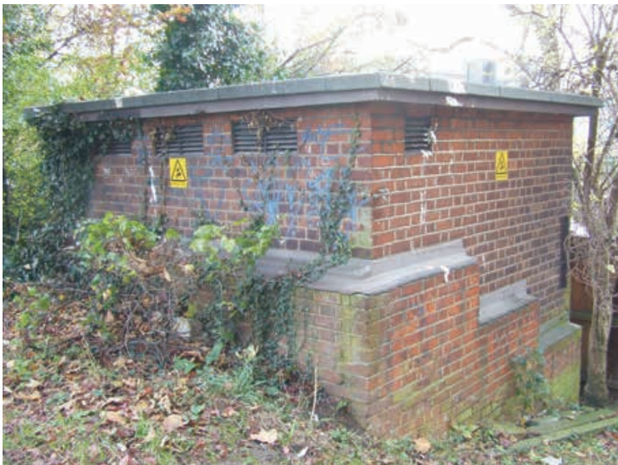
Plate 4: Electricity Sub station at the northwest of site
