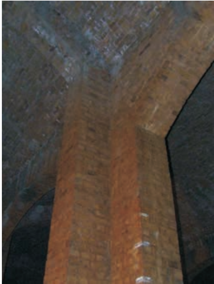
Plate 5: View up at the brick arches within the reservoir
