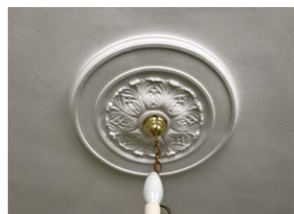
Ceiling Rose (non-original)
