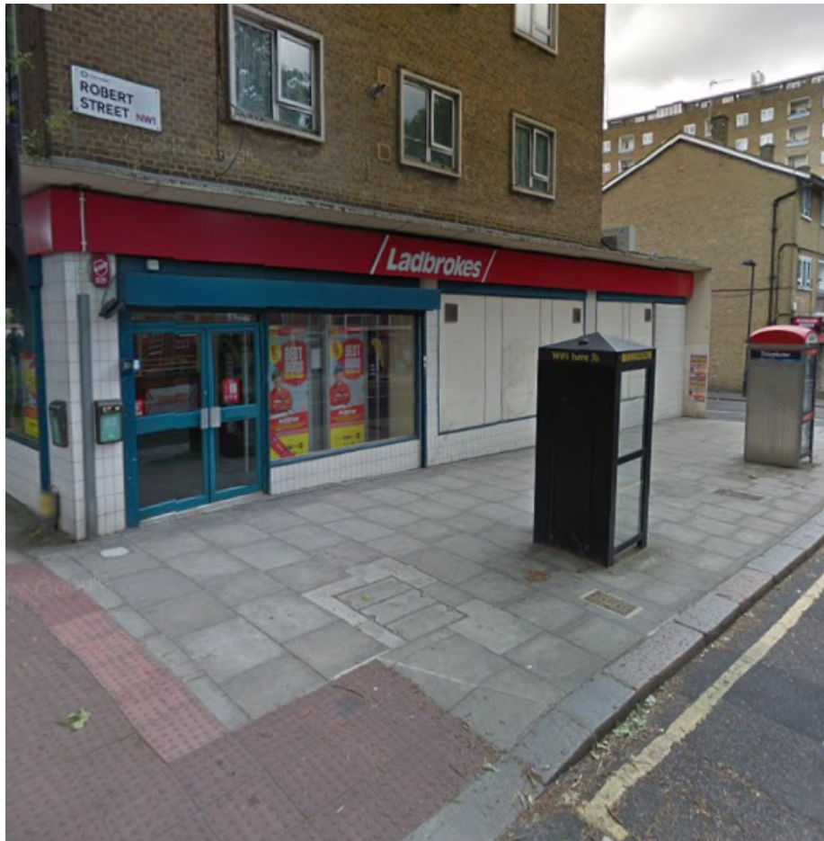
Photo 5: Kiosk at 124 Robert Street, (Jnc Albany Street) (left). To be removed without replacement (secured by Section 278 Agreement). BT kiosk to the right will be unaffected.
