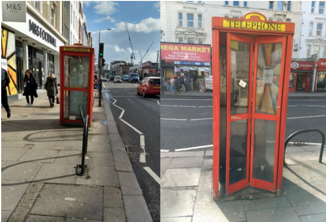
Photos 1 and 2: Existing kiosk outside 72 Kilburn High Road (to be replaced)
