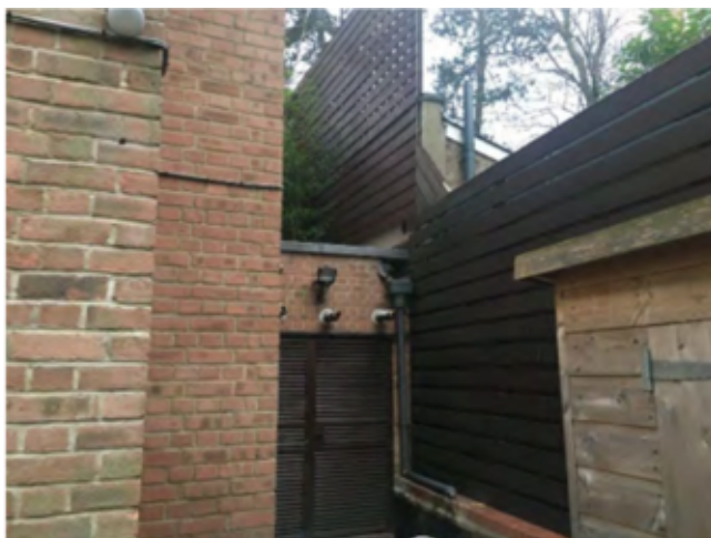
2. Photo showing location of proposed acoustic enclosure at rear of 1 Branch Hill
