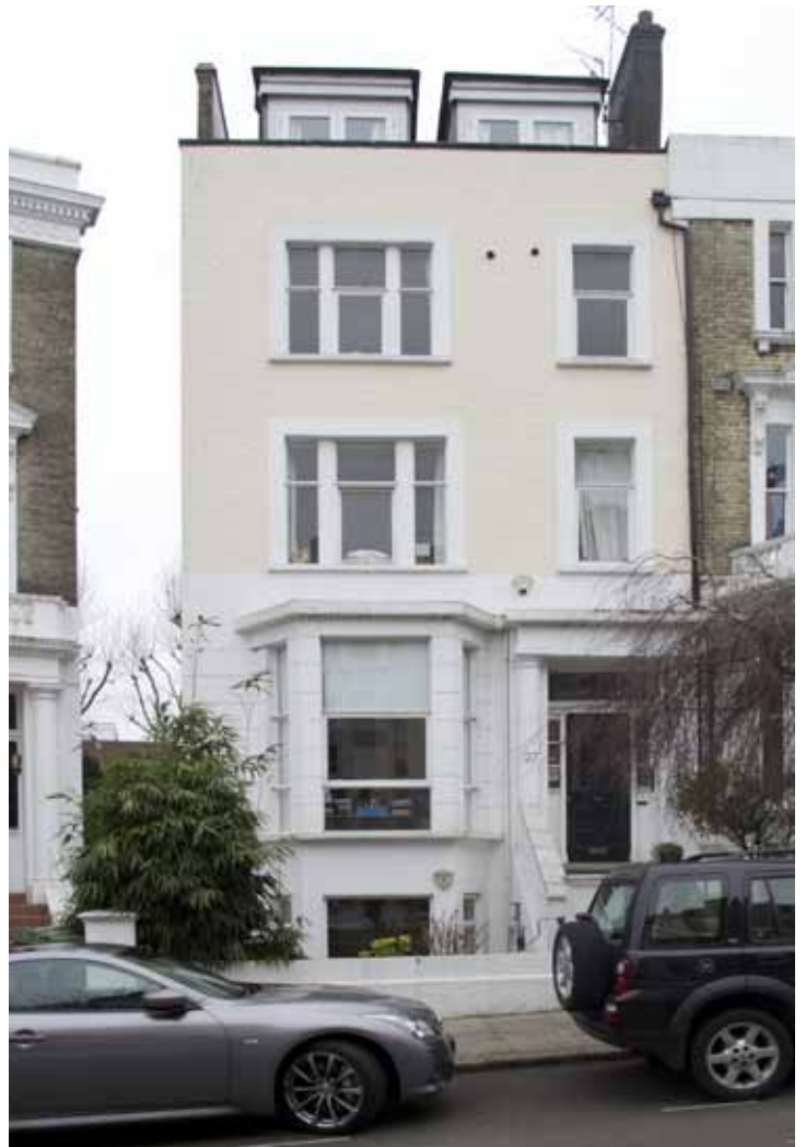
Front Elevation with stripped back detailing and hardlandscaped front. No.27 Belsize Crescent
