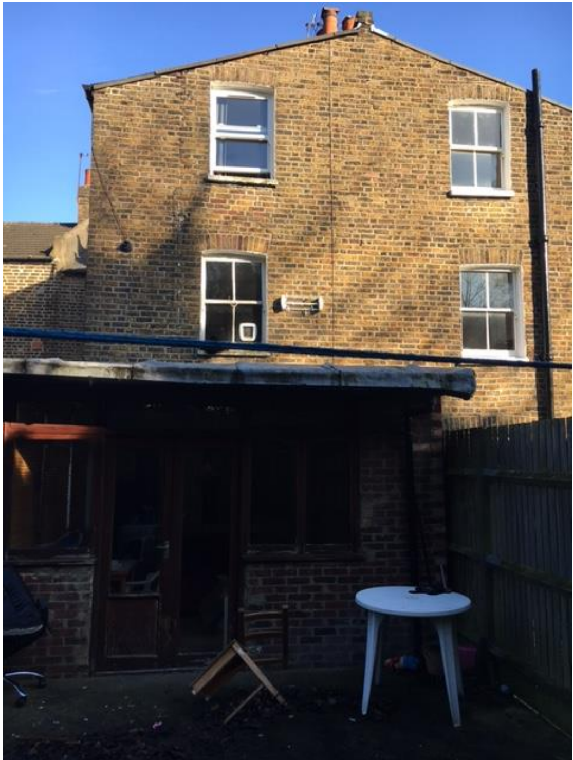
Photo 1- Existing Rear Extension
