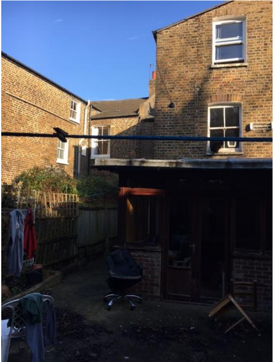
Photo 2- Existing Rear Extension
