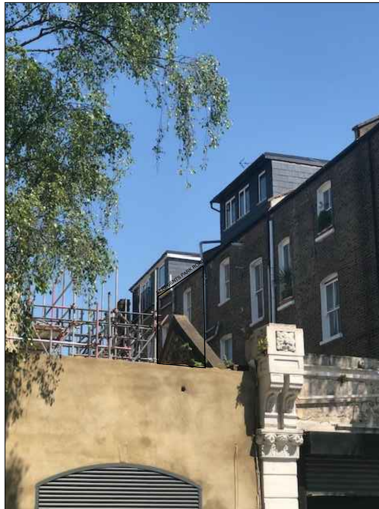
Photo 03 - View of the rear elevation
