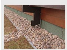
The pebble barrier installed on this project also prevents erosion of the XF301 sedum blanket vegetation from water draining onto the roof from the roof area above via a downpipe.
