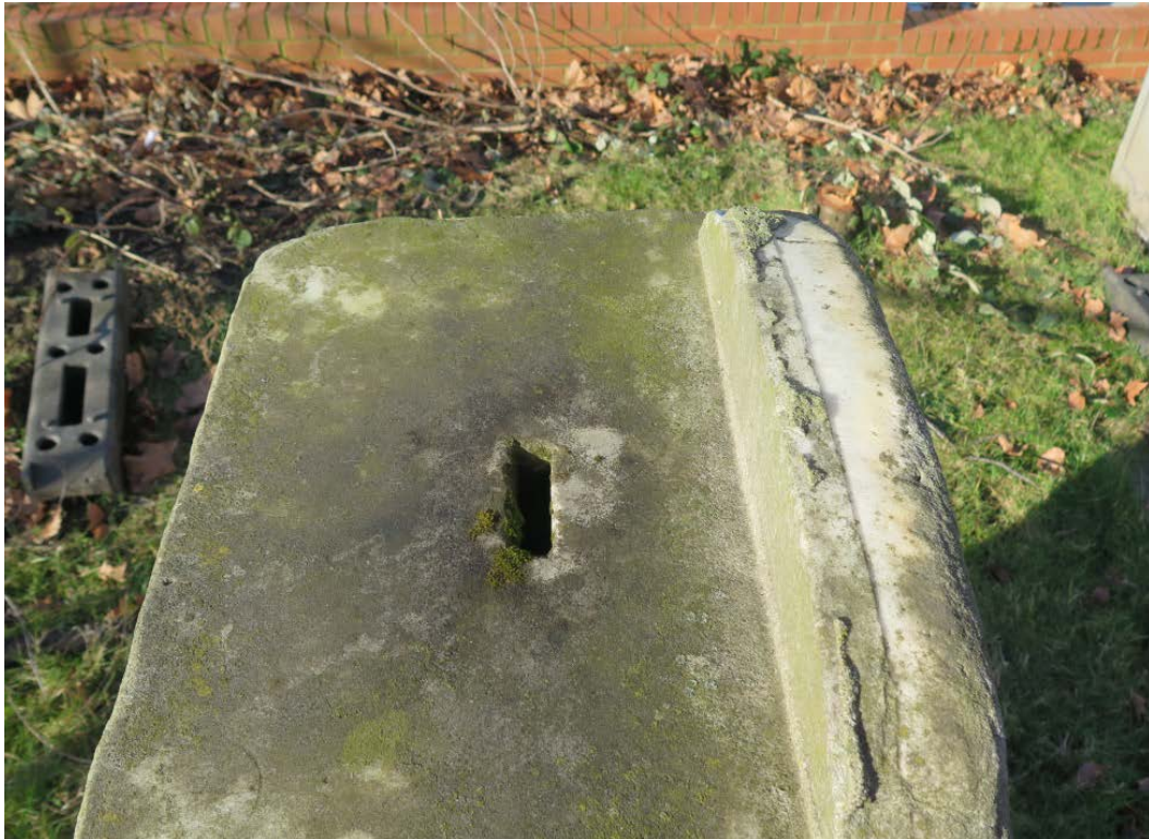
Figure 10 Bird's eye view of top of monument, with probable Lewis pin hole and fixing hole for fallen obelisk
