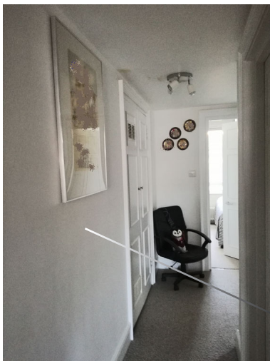
Hallway: service void to be reduced
