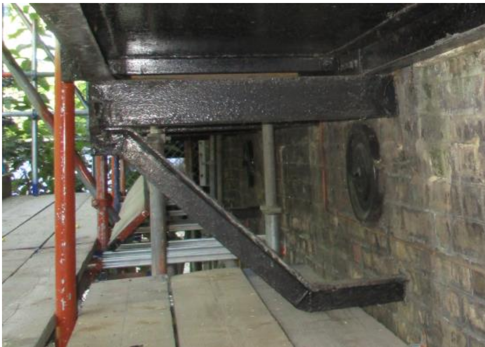
Figure 2 - Example of an existing braced support to the balcony
