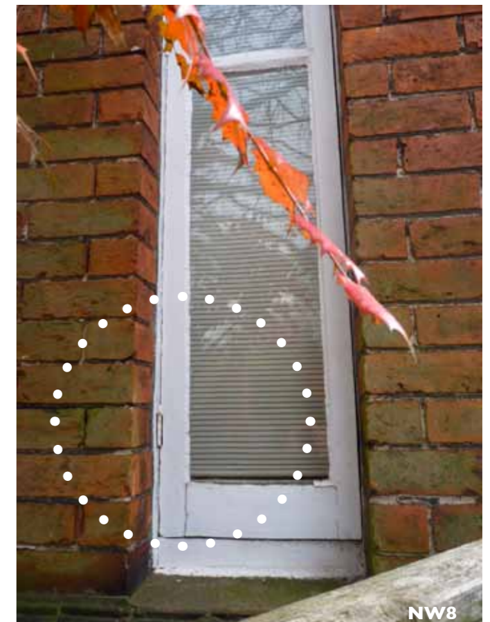
Photo NW8 Circled replacement hinges to some of the casement windows on ground floor of corner bay.
