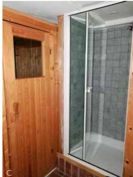
Photos A-C Photo A shows the staircase. Photo B shows new pier column which supports new beam. Photo C shows timber partition between the sauna and shower.
