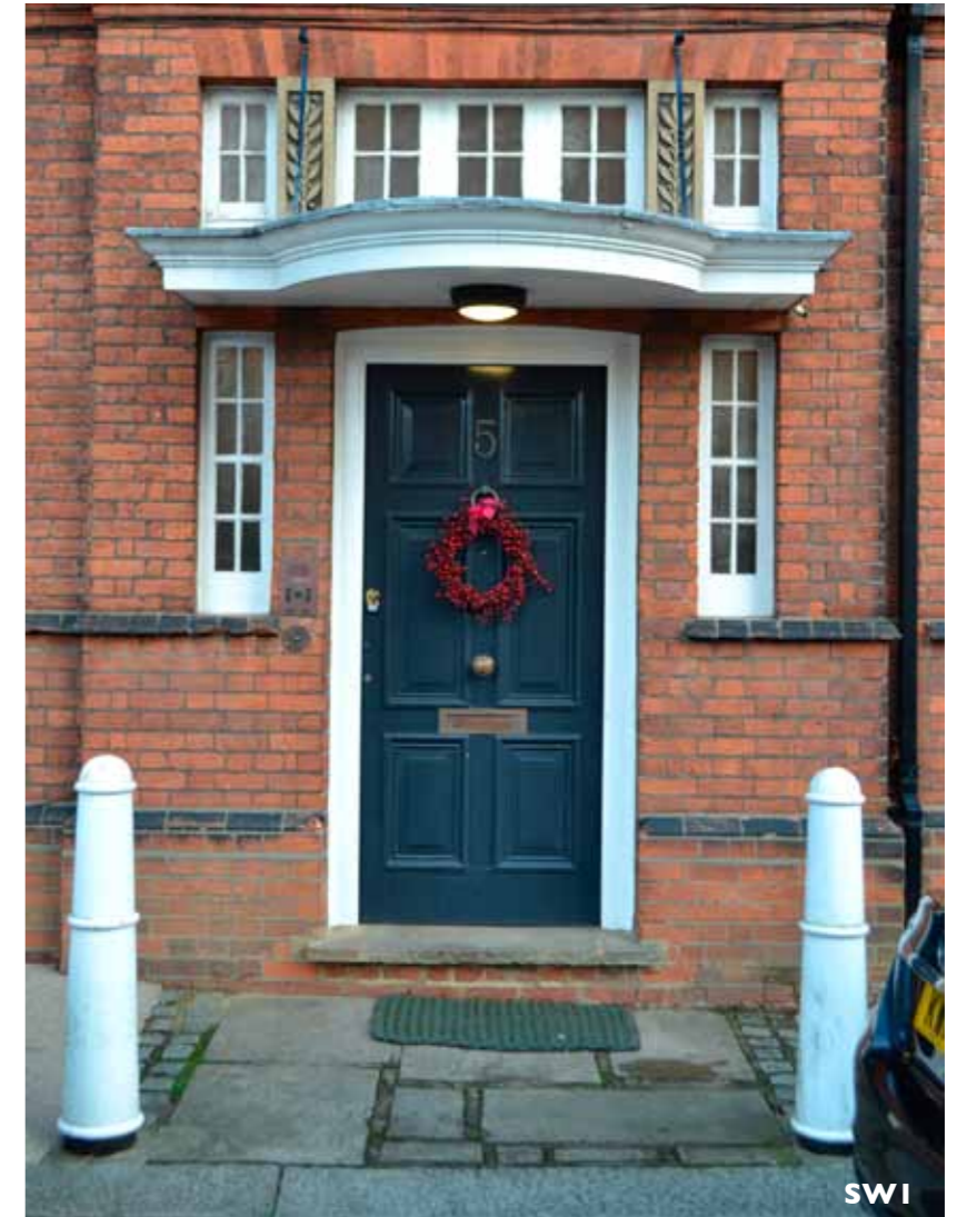
Photo SW1 Existing main entrance on South -West Elevation. The door is relatively modern however the side windows and the fan windows above canopy appear to be original.
