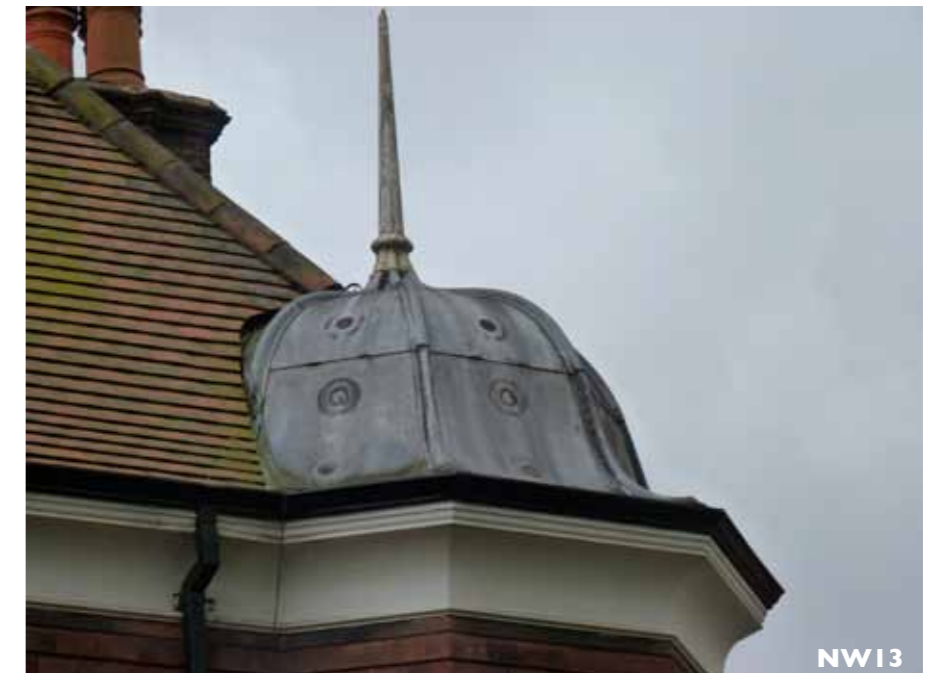
Photo NW12-NW13 Photo NW12 shows gabled two- light dormer with sashes with decorative gable. Photo NW13 shows the ogival leaded roof with tall finial to corner bay.
