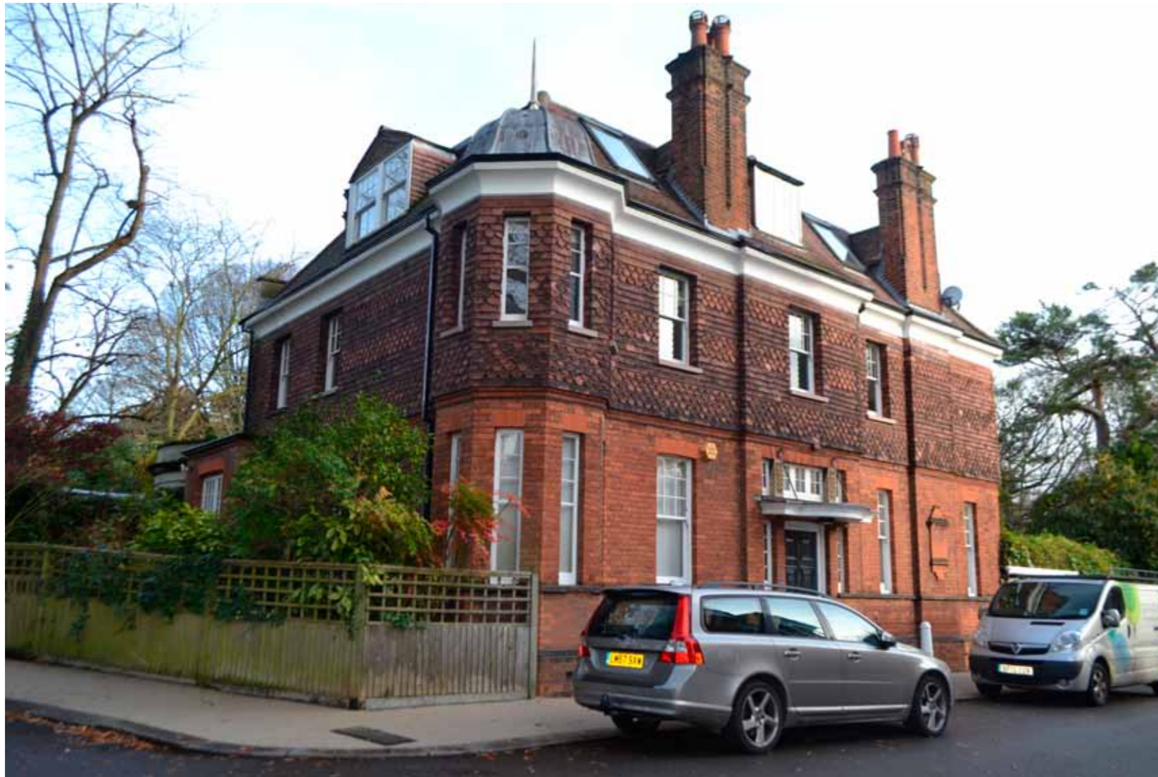
5 Gainsborough Gardens as it exists today
