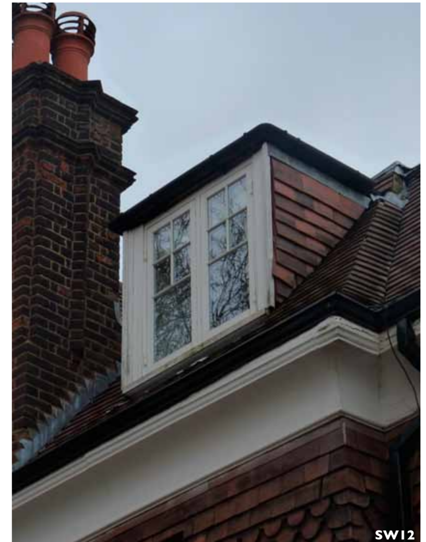
Photos SW10-SW12 Typical windows on second floor of South -West Elevation. The roof lights are relatively new and the dormer window is replacement double glazed casement window.
