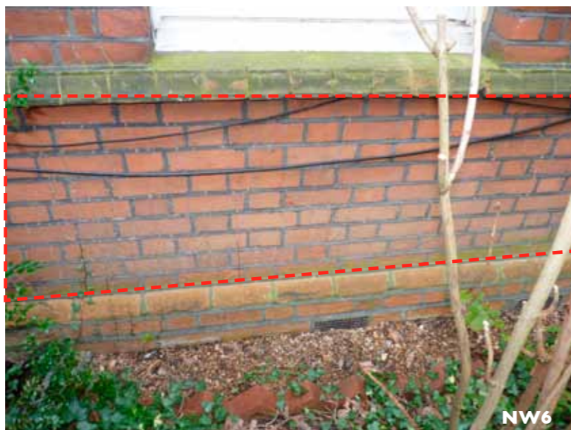
Photos NW5-NW6 Red dashed line denotes the repointing work that was carried out to the ground floor walls. Some of the windows were drought proofed with caulk which is visible on photo NW7
