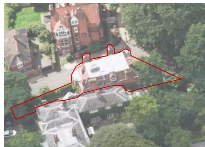
North East aerial view
