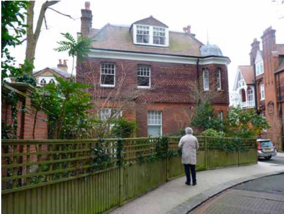
Existing timber fence to the front garden
