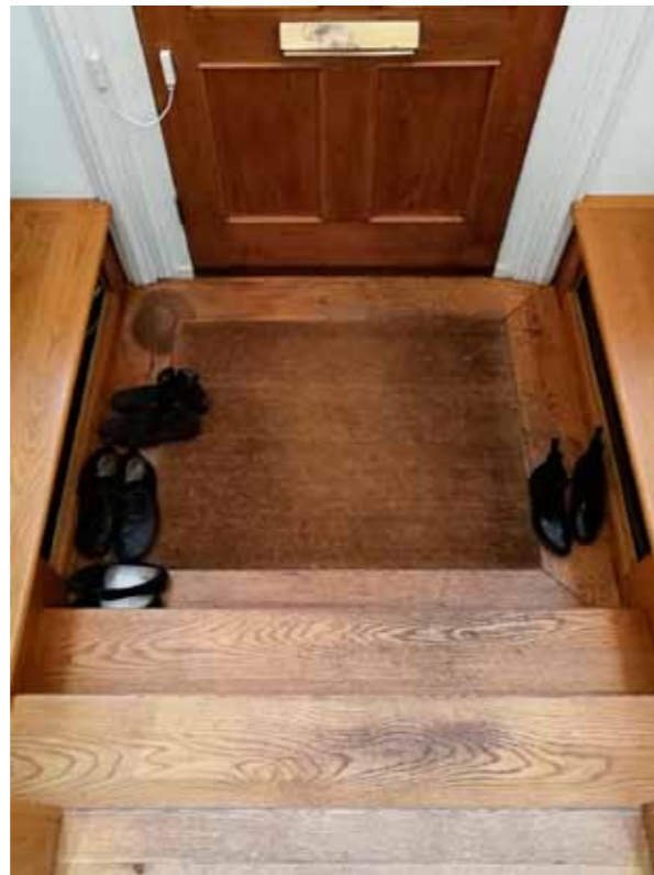
Existing Internal stairs to the front entrance lobby
