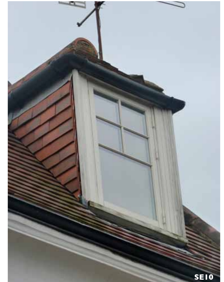
Photos SE9-SE10 Existing second floor dormer windows on South -East Elevation. These are modern timber casement windows.
