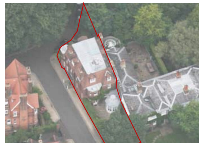
South - West aerial view
