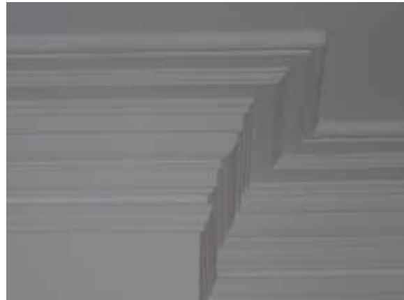
Moulded cornice detail to the ceilings
