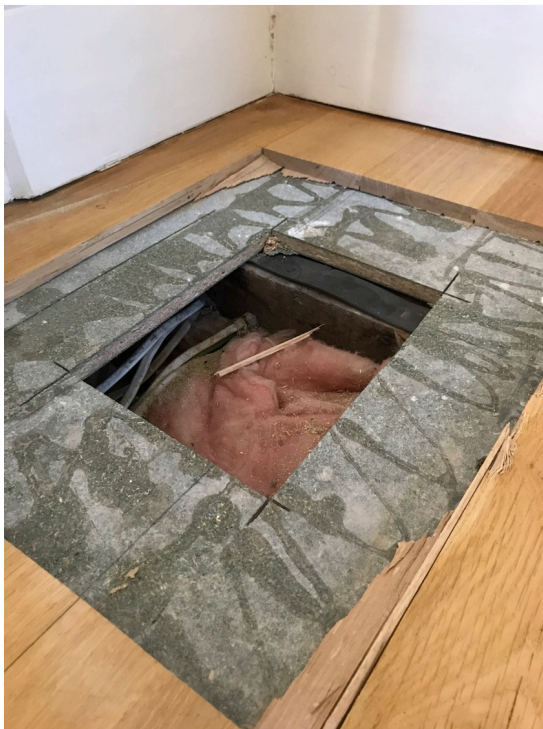
First Floor- Existing Floor Materials- 18mm non-original floorboards, 18mm chipboard
