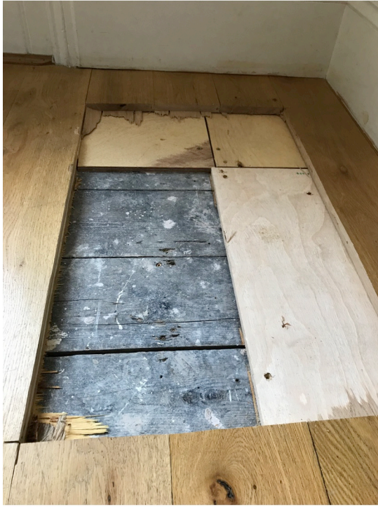
Ground Floor- Existing Floor Materials- 18mm non-original floorboards, 12mm plywood, older floorboards
