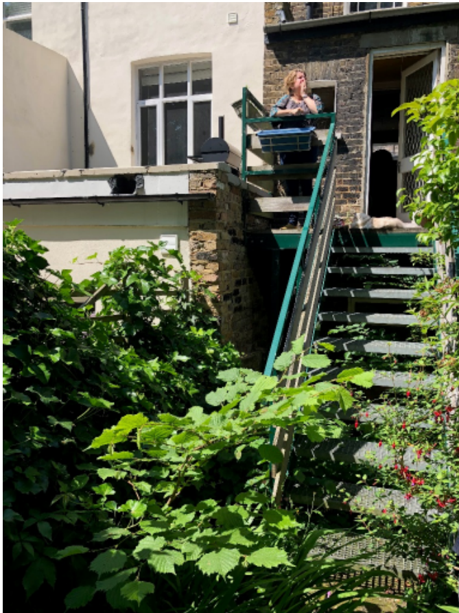
6. View from 34 Burghley road showing relationship between extension and existing balcony
