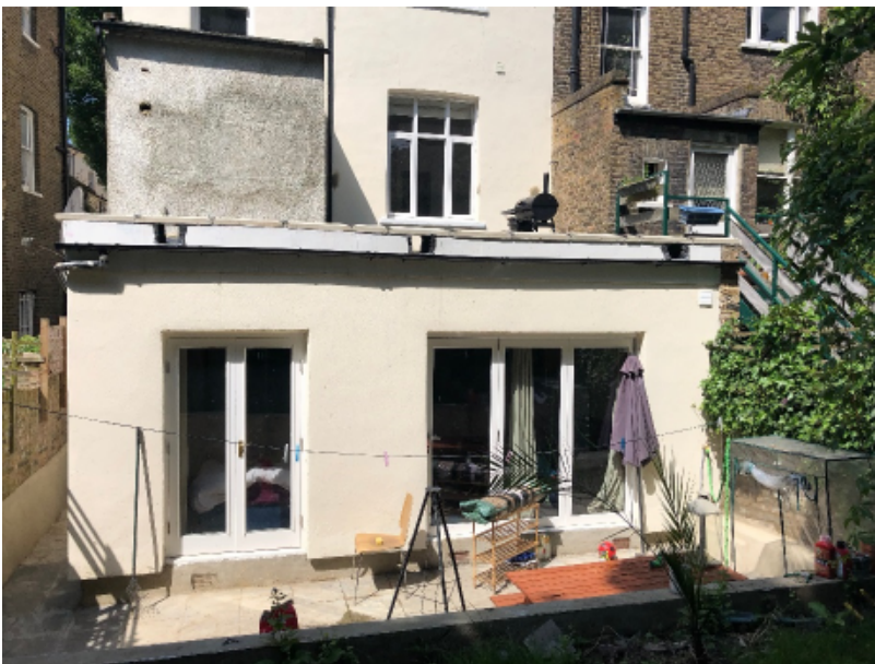
2. View towards rear elevation of 32 Burghley Road (above) showing lower ground floor extension and upper ground floor extension
