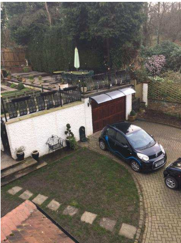
Existing Garage and Retaining Structures
