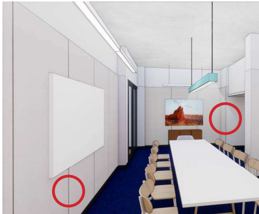
FABRIC GAP CLADDING AND FABRIC EDGE (EXPOSED OR CAPTURED)
