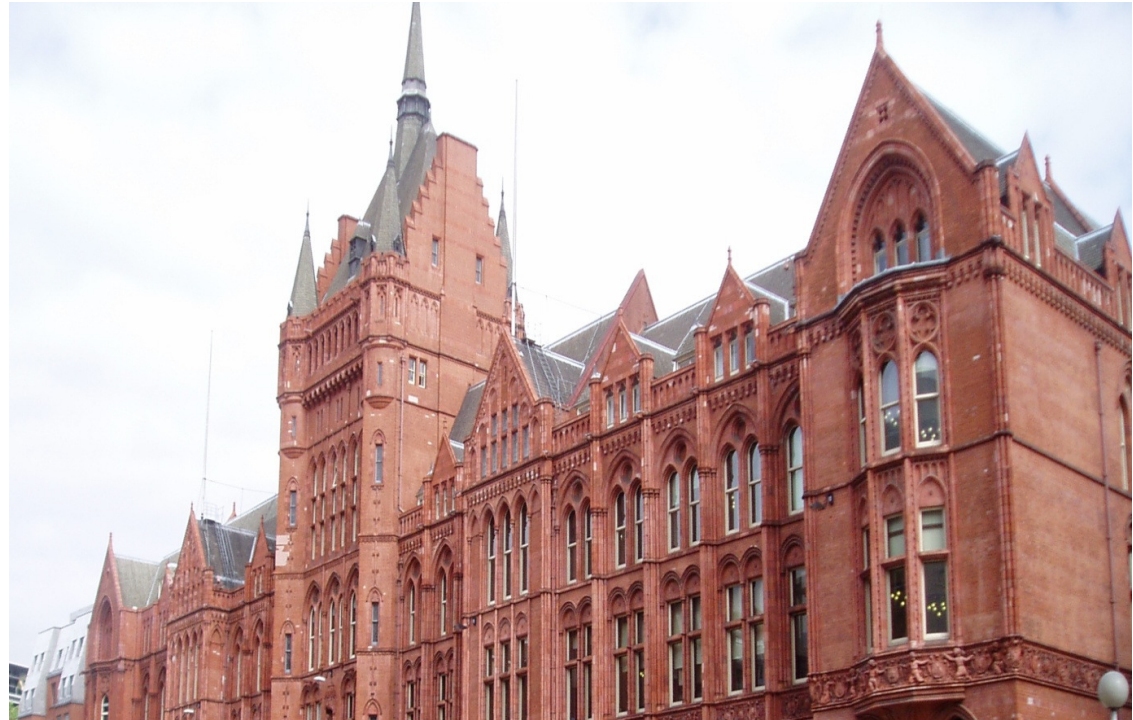
Waterhouse Square’s impressive frontage onto High Holborn
