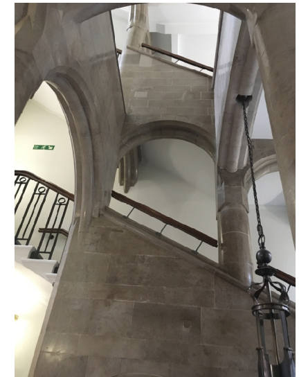
South West staircase
