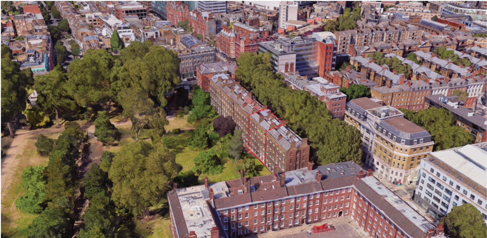
AERIAL VIEW OF 2 VERULAM BUILDINGS
