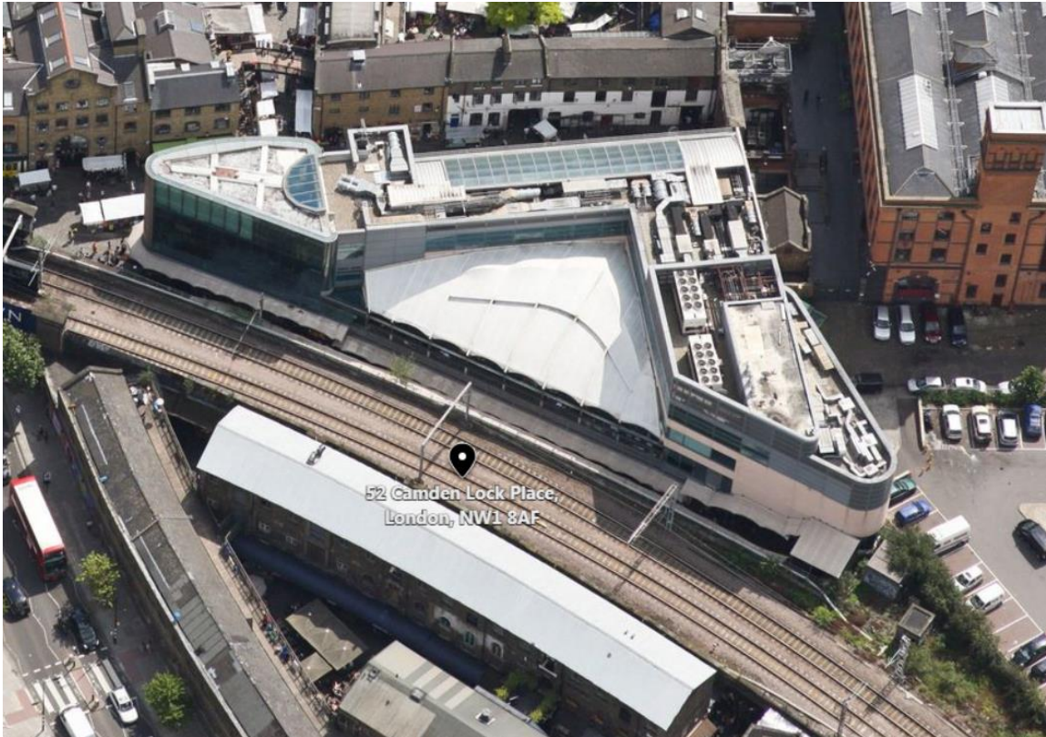
Photo 3: Aerial view of north elevation
