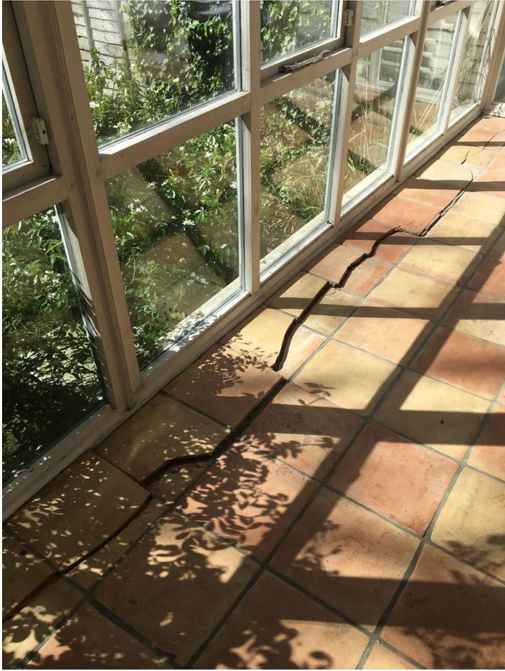
Sunken floor in living room, this needs repair in order to maintain the structural integrity of the building.
