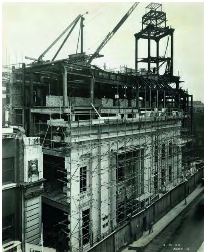
Figure 6: Great Queen Street elevation in construction c1930 (©UGLE)
