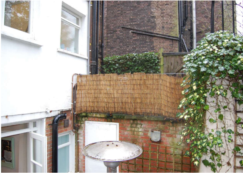
View of existing meter room from existing Patio
