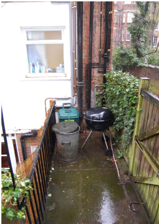
View of existing Meter Room Roof
