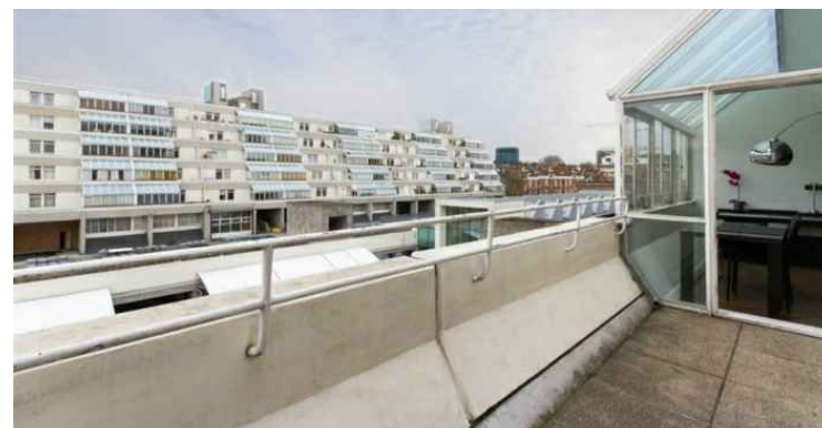
[05] PRECEDENT IMAGES (BRUNSWICK CENTRE FLATS BALUSTRADE)
