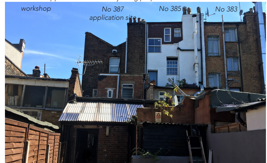
Rear view of application site and adjoining properties
