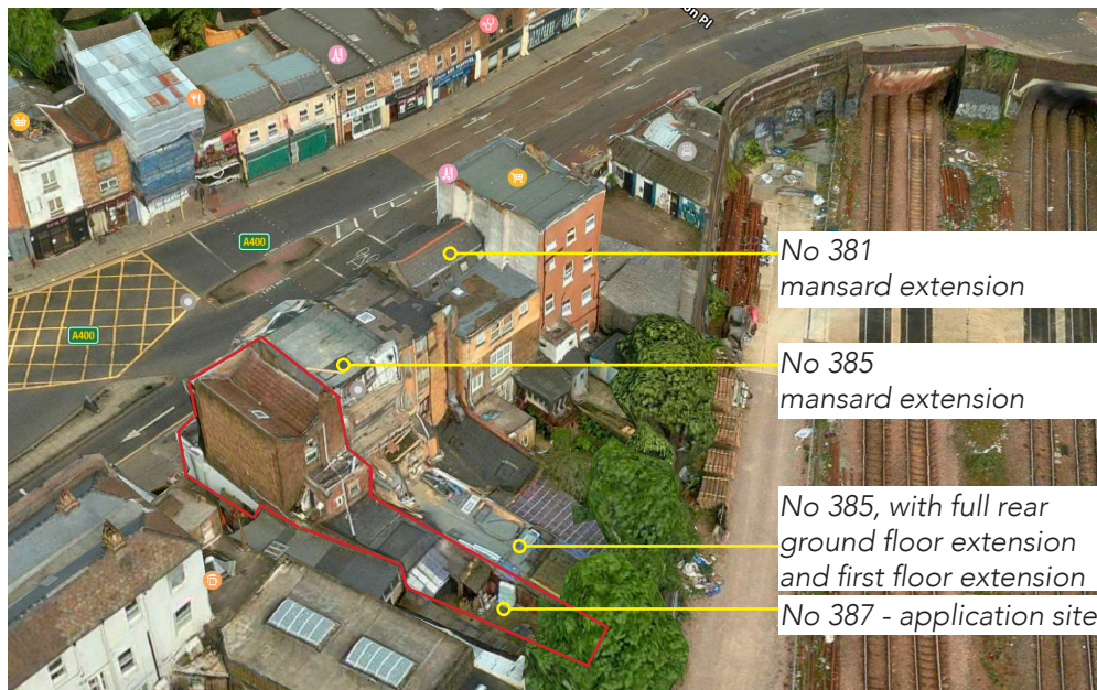
Aerial of the rear of the application site and neighbouring properties
