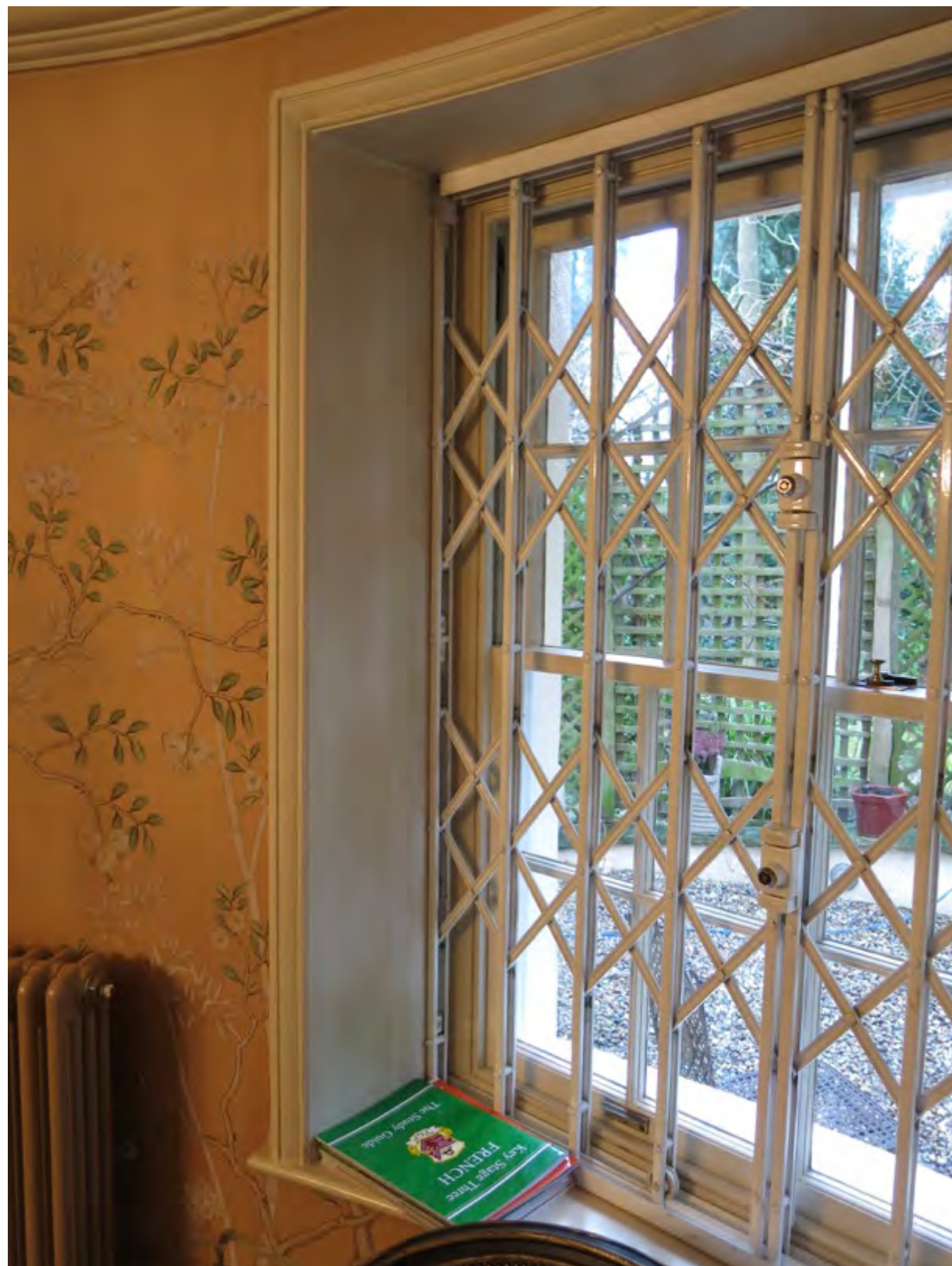
Figure 30: The timber lined sash window reveal
