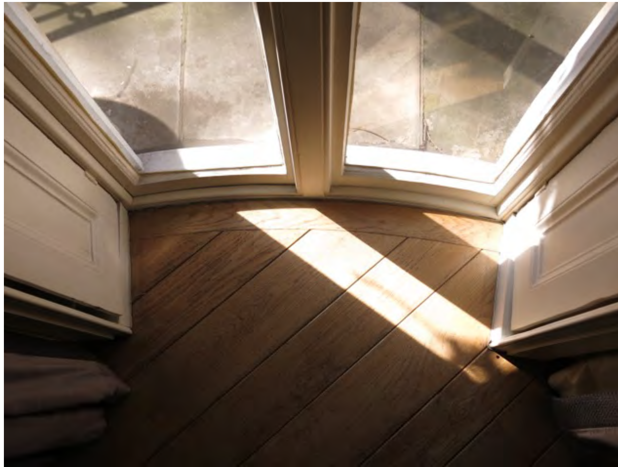
Figure 26: View looking at the internal window recess, cill and shutters
