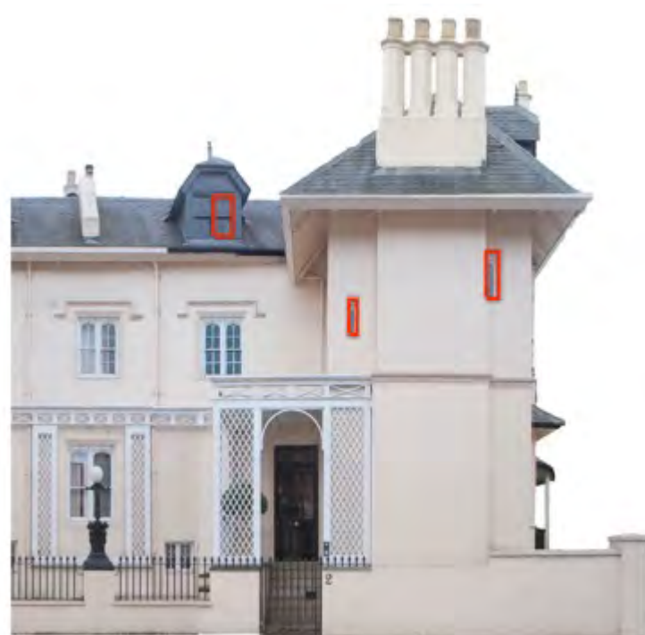
Figure 9: A view of the east elevation of 2 Park Village East. Windows where internal secondary glazing will be installed are annotated in red
