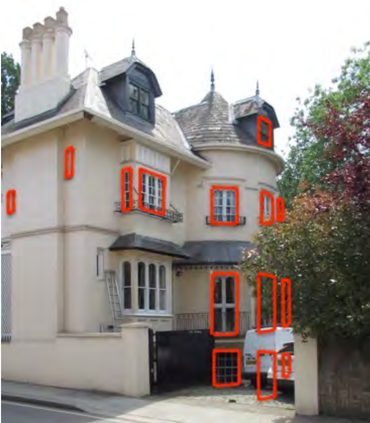
Figure 10: A view of the north elevation of 2 Park Village East. Windows where internal secondary glazing will be installed are annotated in red.
