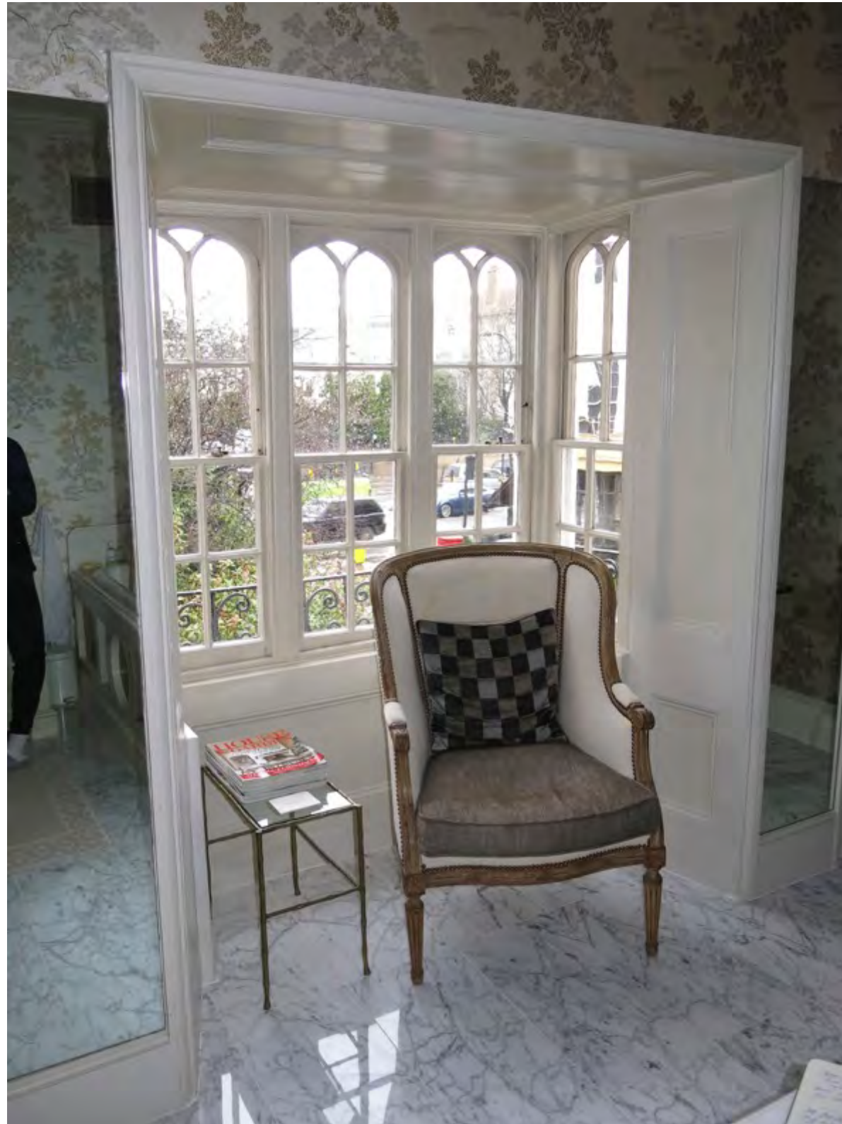
Figure 18: View of the original sash window bay facing north. Secondary glazing will be installed internally in the entrance to the bay window
