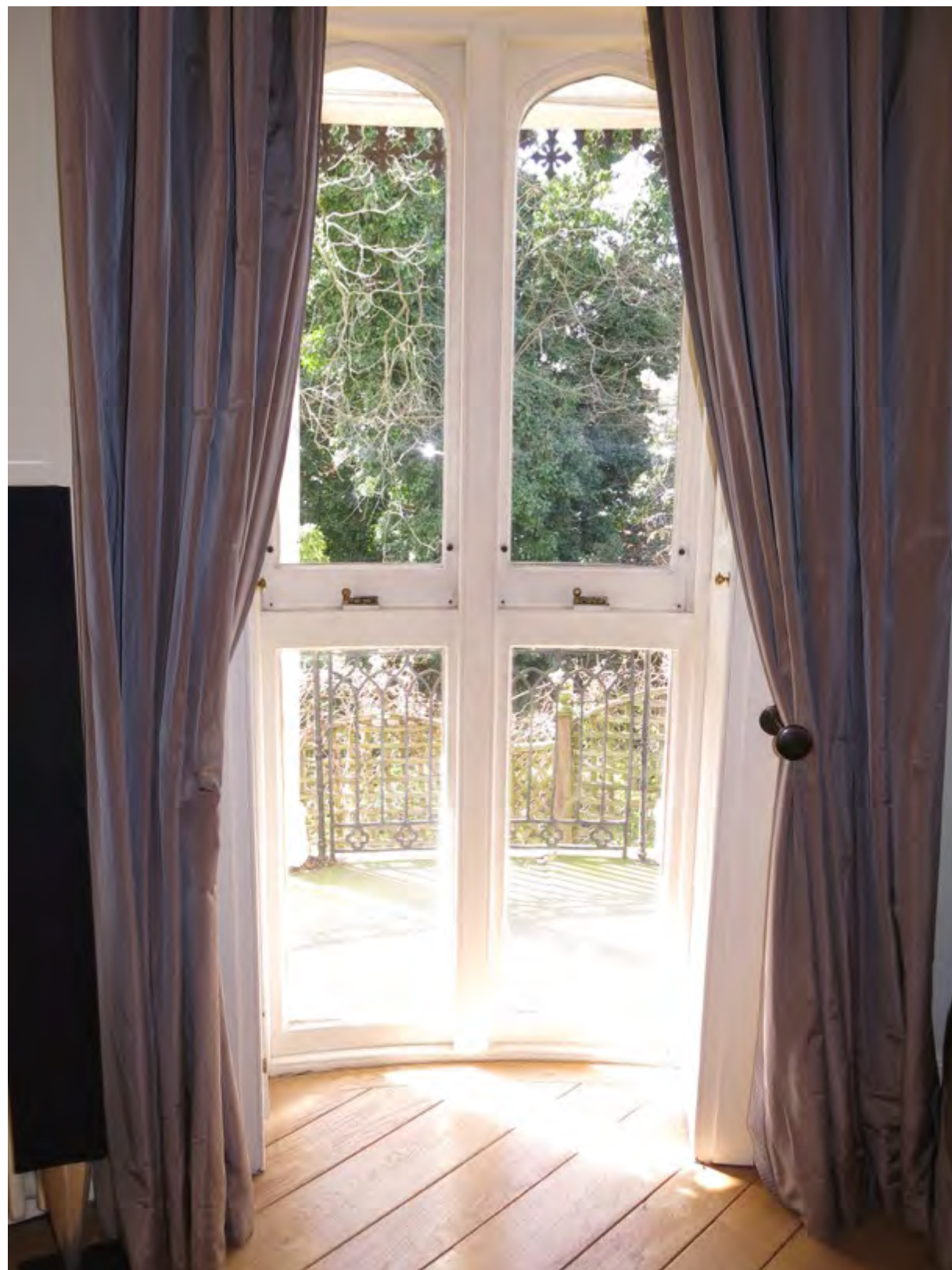
Figure 24: Typical internal window elevation with a pair of full height sash windows
