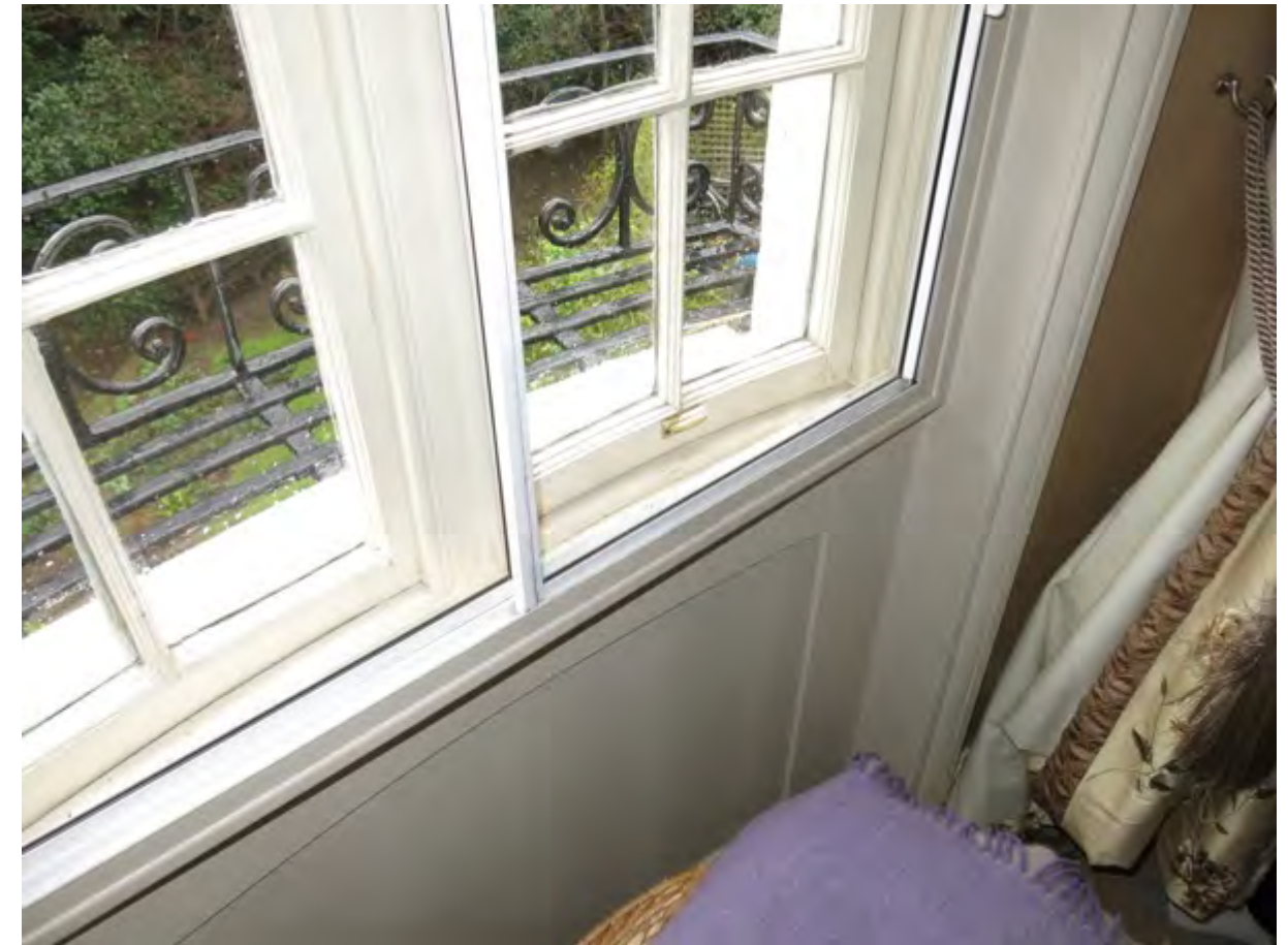
Figure 17: View of the existing internal window cill with secondary glazing. Note; the original sash window is curved in plan
