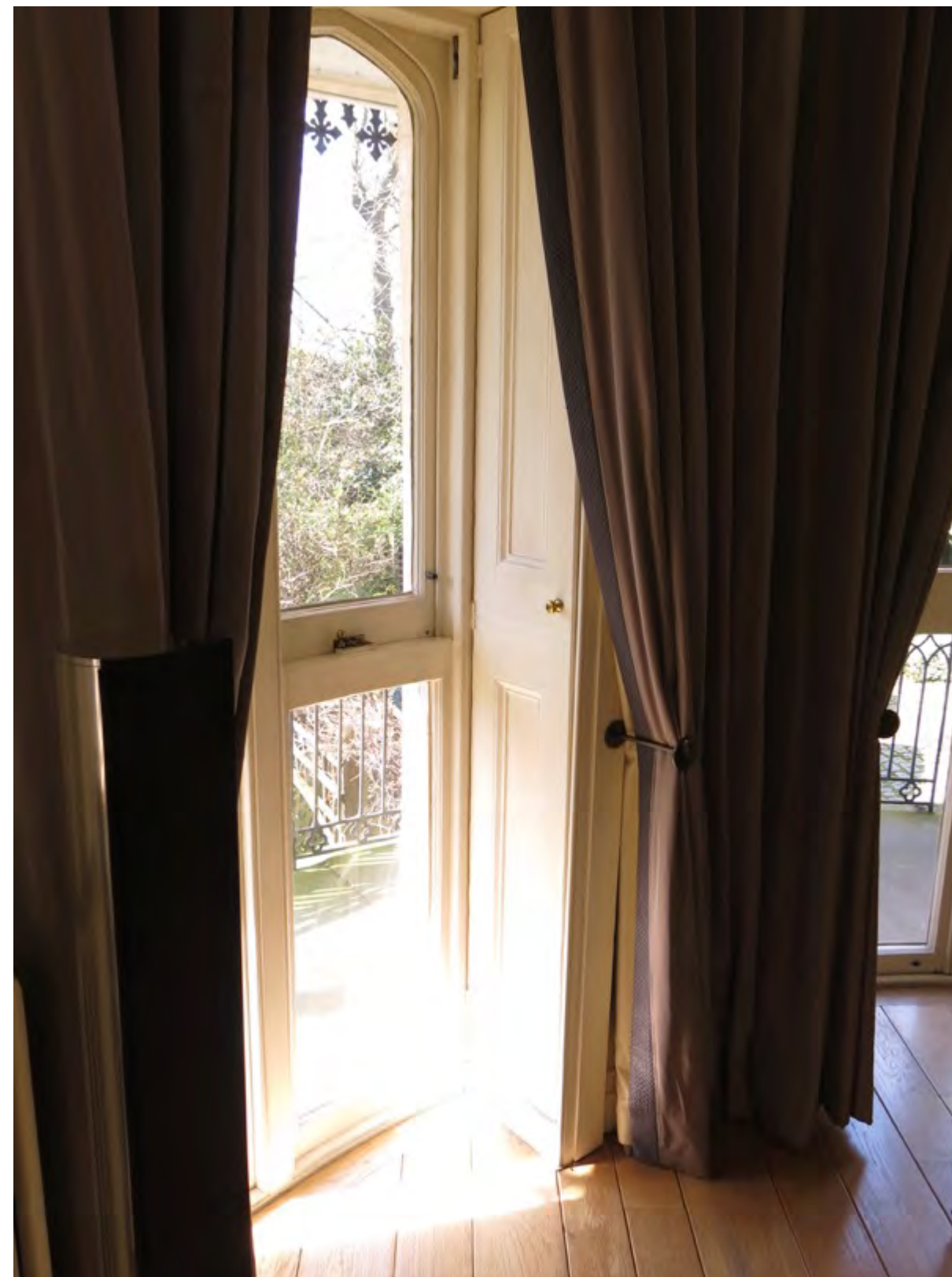
Figure 25: Sash window with shutters folded back to create a panelled window reveal. Secondary glazing will be temporarily fixed to the shutters which will remain inoperable whilst the glazing is installed. Secondary glazing will be removed on completion of the HS2 construction works and the shutters will be restored to operational use
