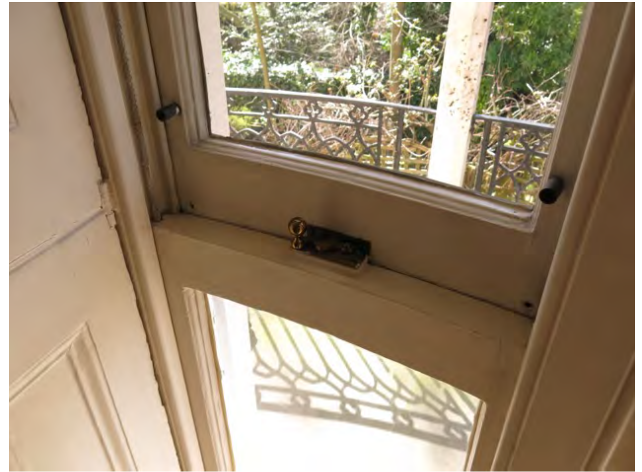
Figure 27: View of the sash meeting rail
