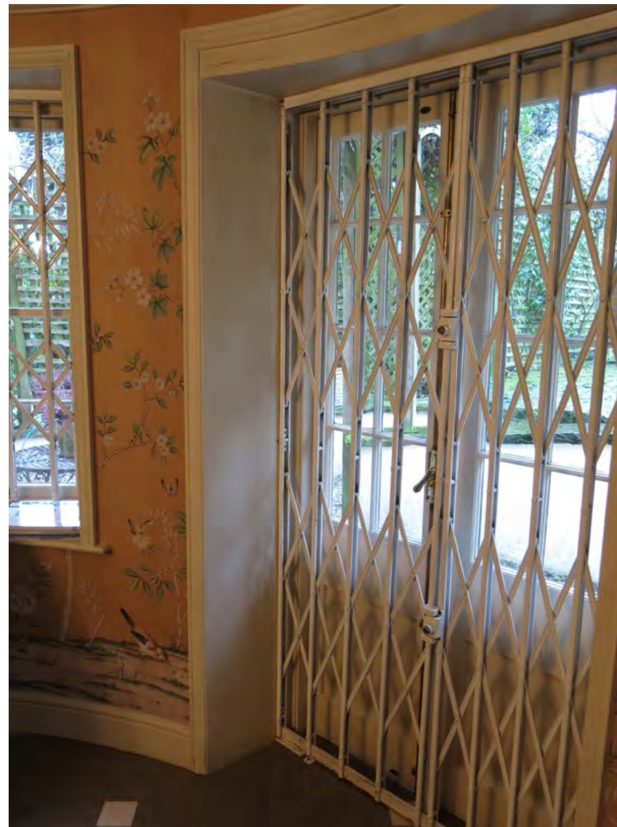
Figure 31: The French door illustrating the reveal depth and existing security grills. An inward opening full height secondary glazing door will be installed within the existing reveal
