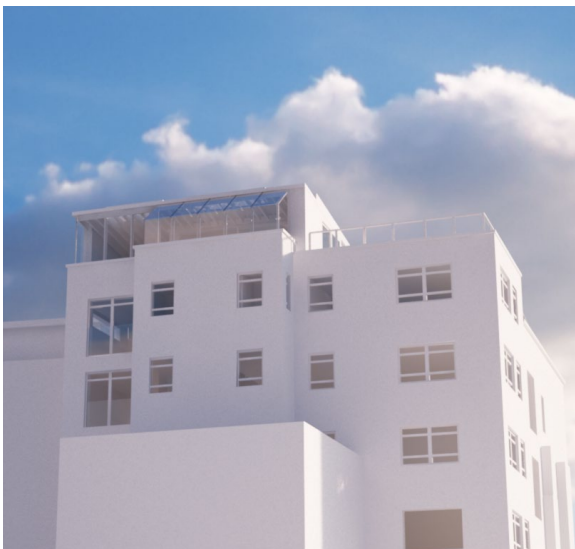
View from cliff Villas
