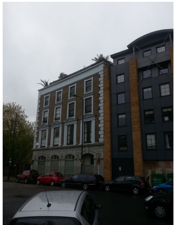
View from York Way looking south
