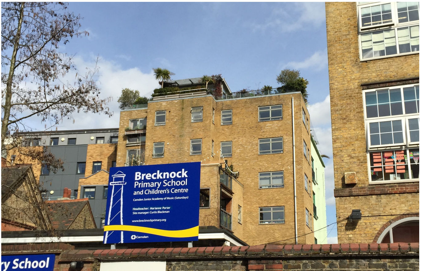
EXISTING VIEW FROM CLIFF VILLAS TO SOUTH
