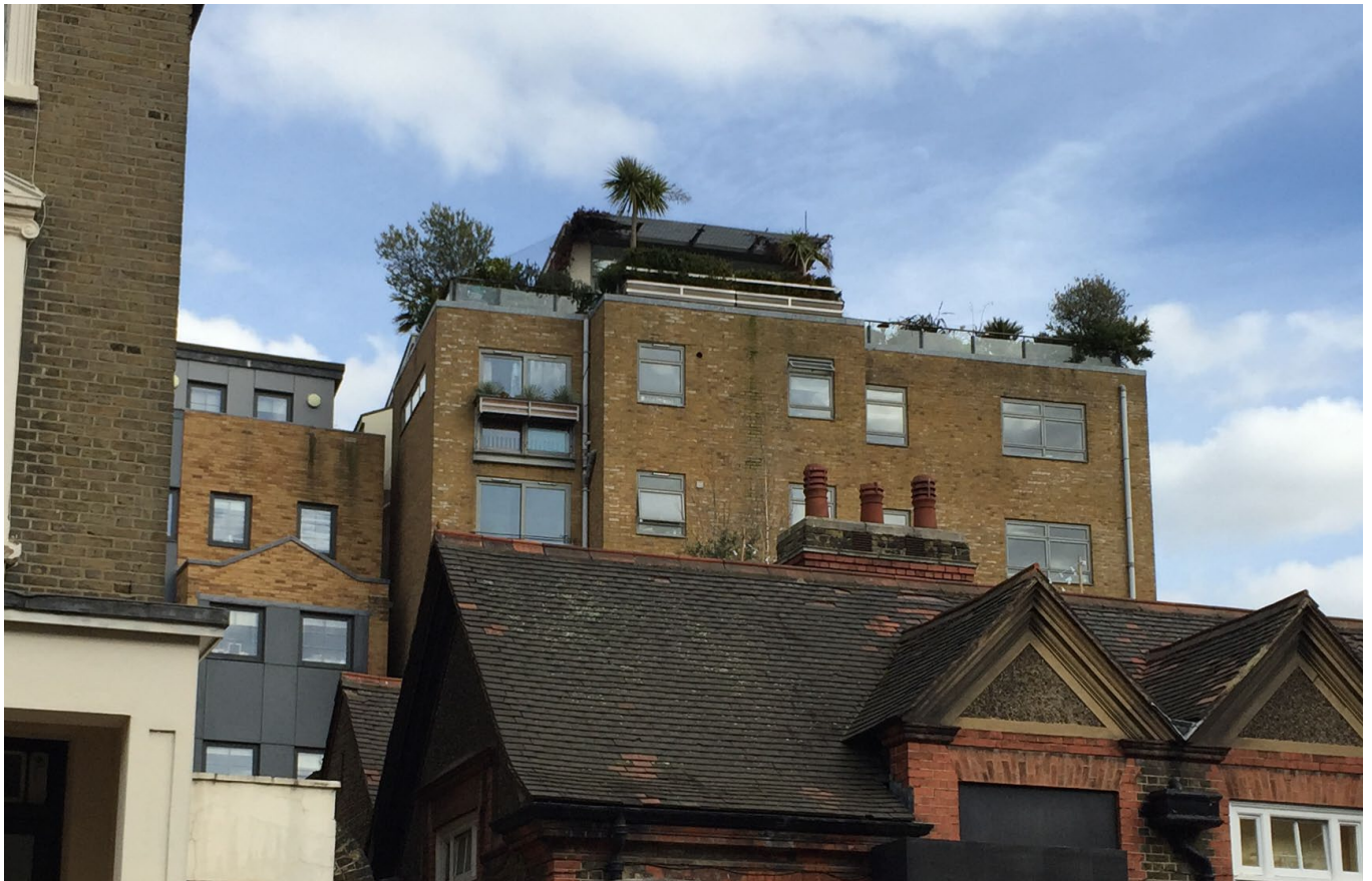
EXISTING VIEW FROM CLIFF VILLAS TO NORTH
