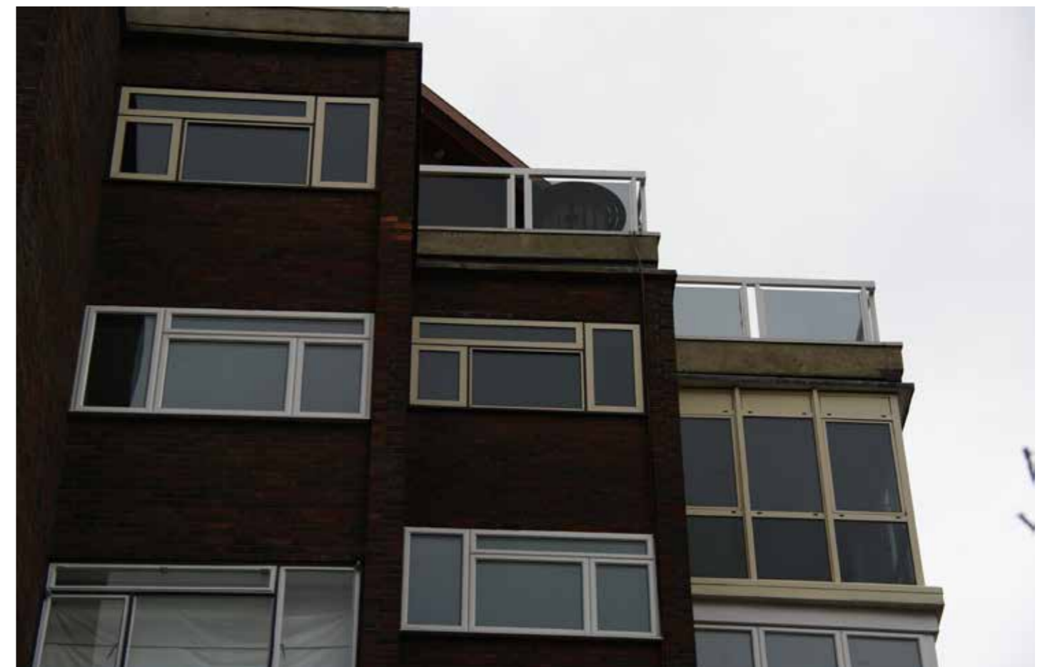
Existing Site Photograph
