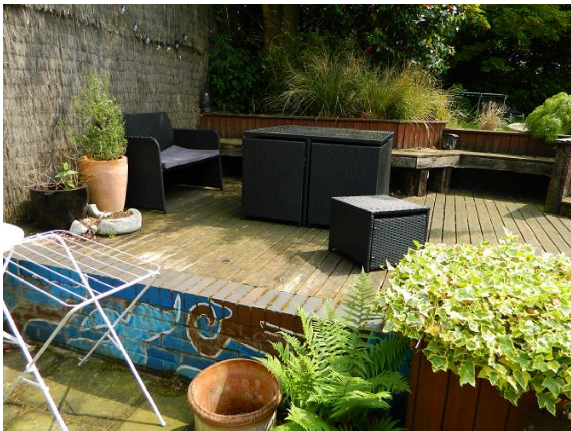
Figure 3. Wooden decking adjacent to T4 which includes two level changes, each with a masonry retaining wall which will serve as a partial root barrier.
