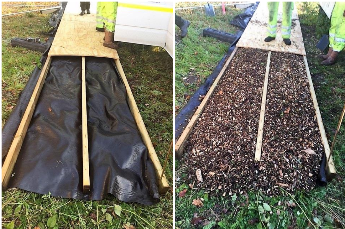
Figure 11. Plywood sheeting used as ground protection.
