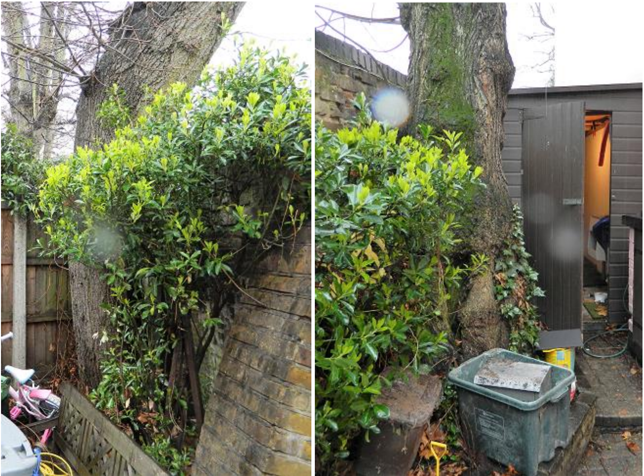
Figure 1. Photographs of lime trees T1 (left) and T2 (right) in the front garden adjacent to the boundary wall.
