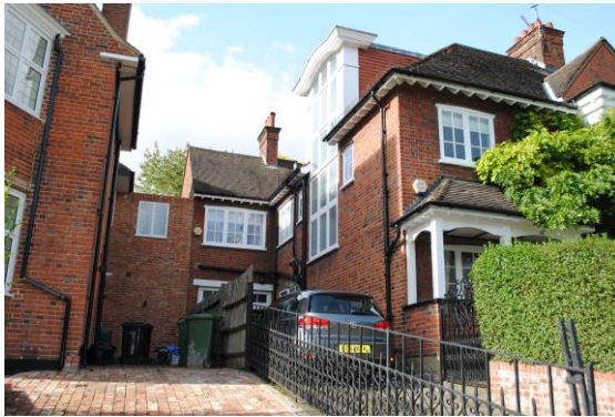
Image: No. 82 Lawn Road, two storey side extension
