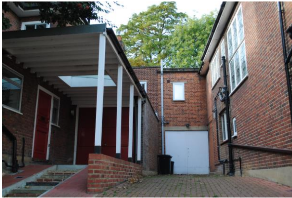
Image: Existing side extension (nos. 75 and 76 Lawn Road)
