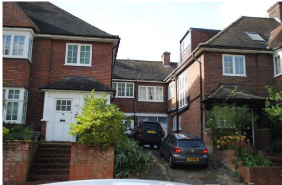
Image: 73 and 74 Lawn Road -two storey extensions
