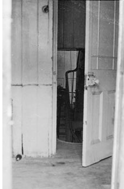
Figure 19: Internal door at Nos. 64/65 Guilford Street, 1980s
