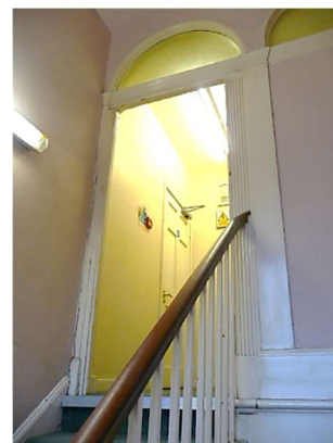
Figure 12 No64 2 nd Fl stair screen
