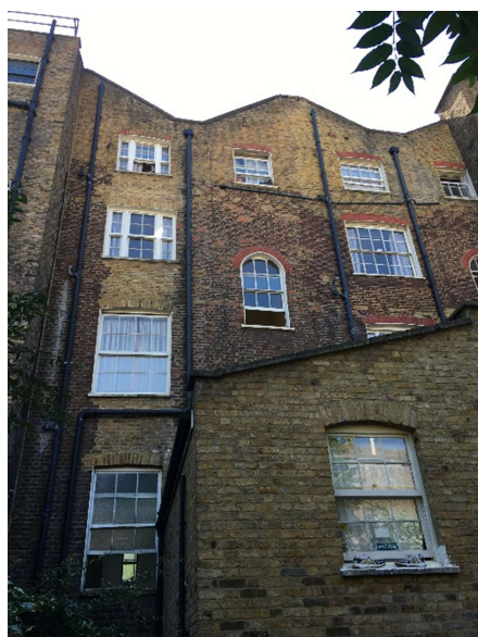
Figure 2- Rear elevation repairs
