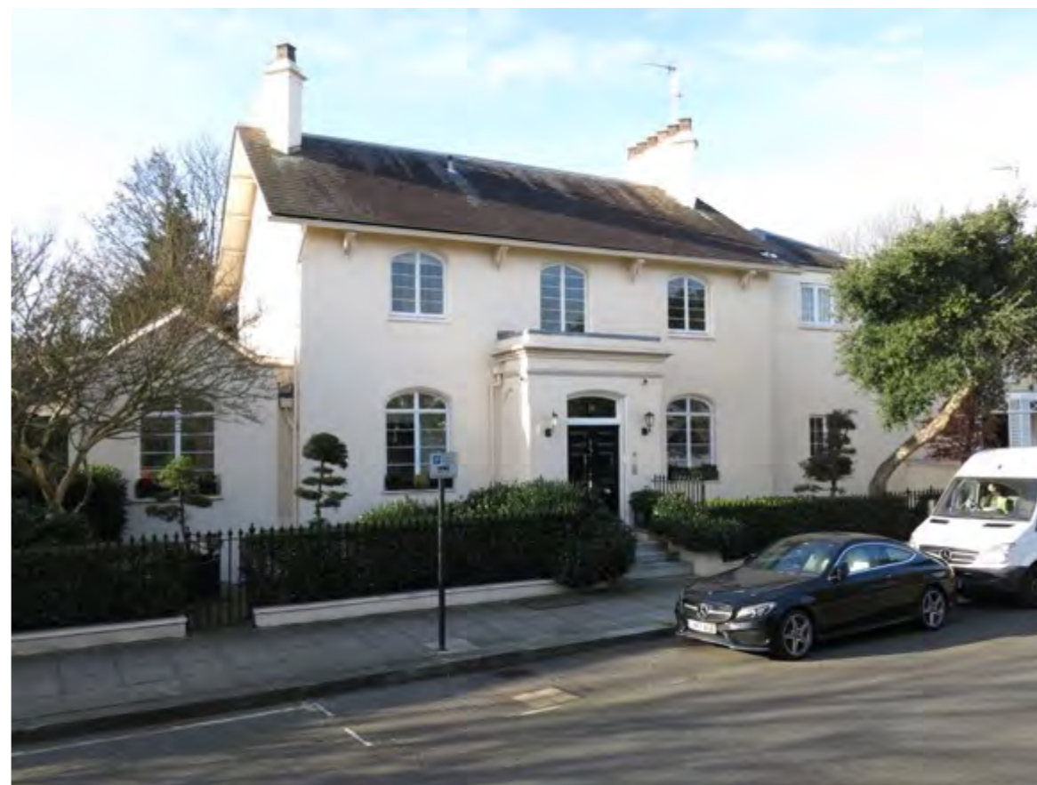
Figure 8: A view of 14 Park Village East taken in February 2018. The photograph illustrates the later extensions to the house creating a two storey addition on the right and single storey addition on the left.
