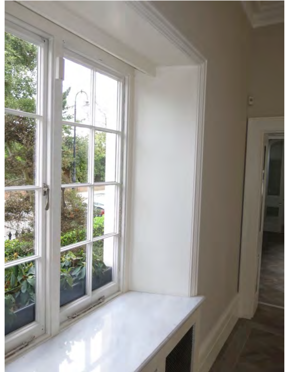
Figure 13: Internal view of the existing casement with spayed timber reveals
