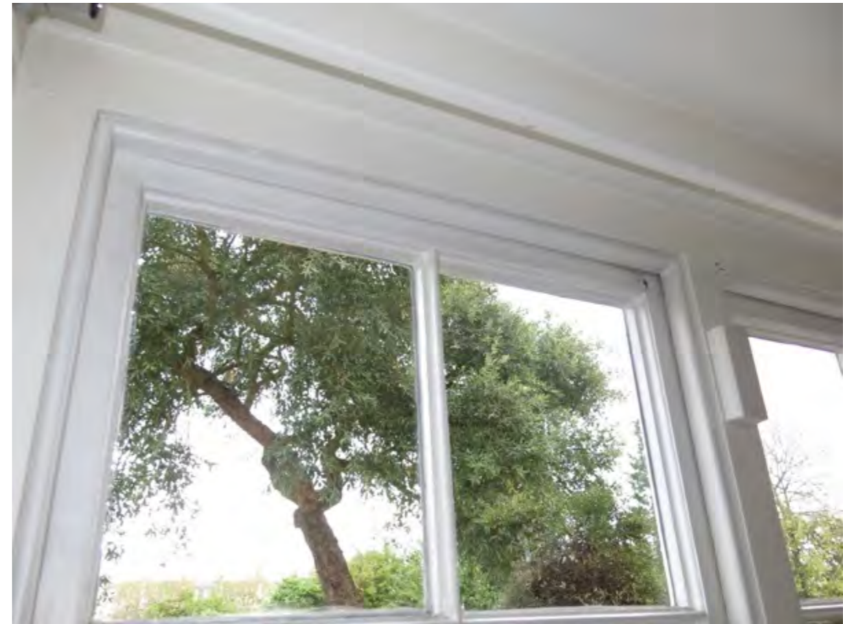
Figure 15: View of the existing casement frame and outward opening casements
