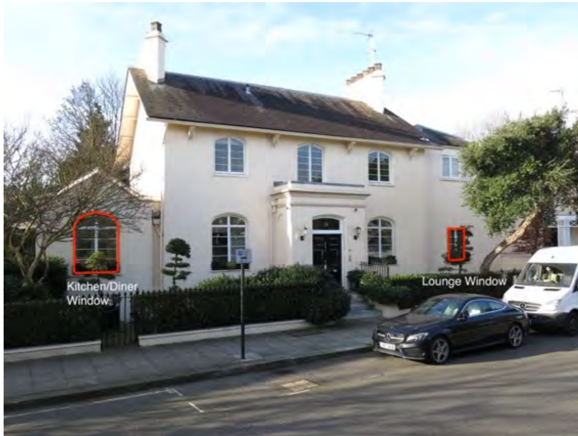
Figure 9: A view of 14 Park Village East. Windows where internal secondary glazing will be installed are annotated in red.
