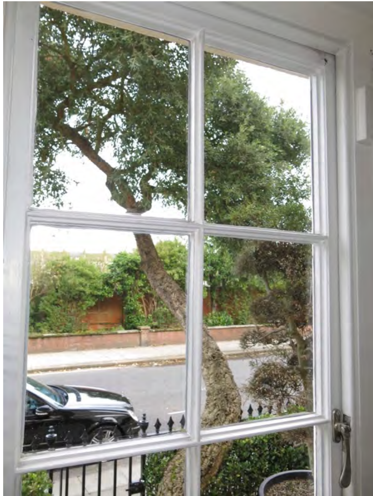
Figure 14: Detail of the existing window casement with moulded timber glazing beads. View looking out onto Park Village East
