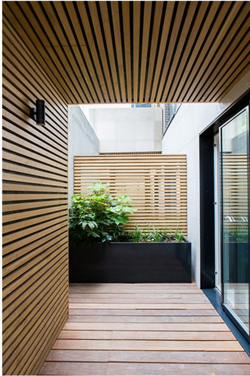
Examples of Western Red Cedar used on trellis and to form external partitions at River Street Mews by Tasou Associates.
