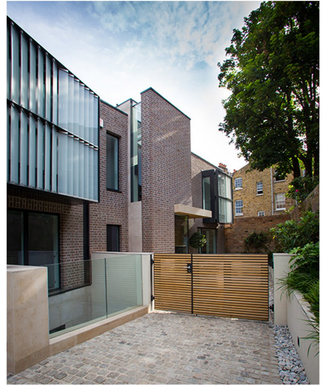
Western Red Cedar infill on pedestrian/vehicular gate, also at River Street Mews.
