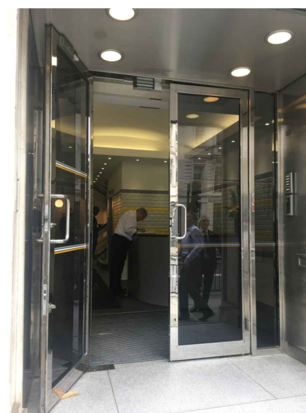
01 Photographs of existing entrance 10.200 1:50@A3
