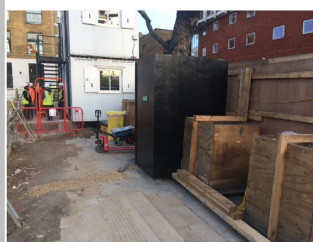
Robust hoarding and temporary concrete ground protection
