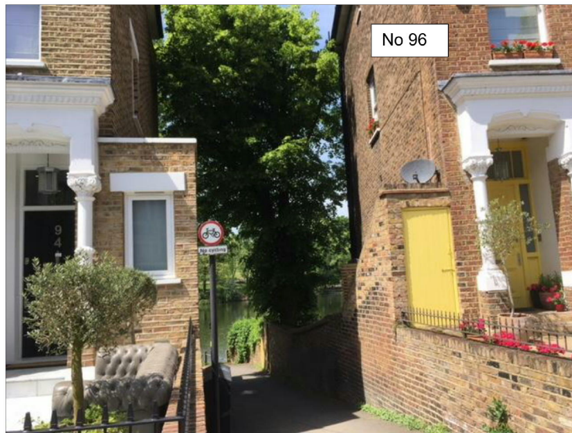
Fig. 1 View of 96 South Hill Park, looking west, with Lime tree T1
