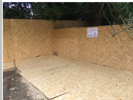
Tree protection Hoarding and ground protection over sharp sand.
