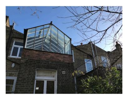
The rear projection has been extended up to a parapet and a conservatory added. This is fully glazed, including the wall to the adjacent property. Note section of poorly matching masonry below conservatory.
