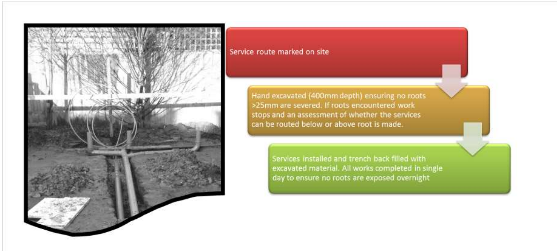
Fig 7 – Service installation overview.
