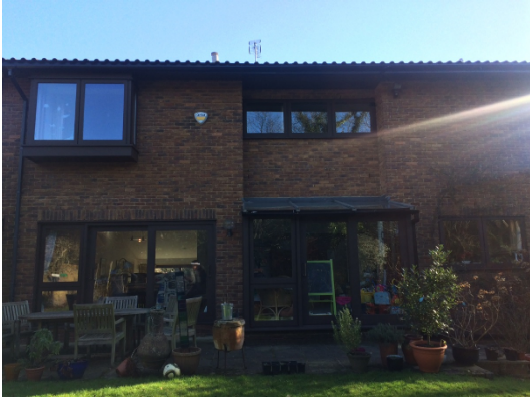
5. Rear elevation of application site
