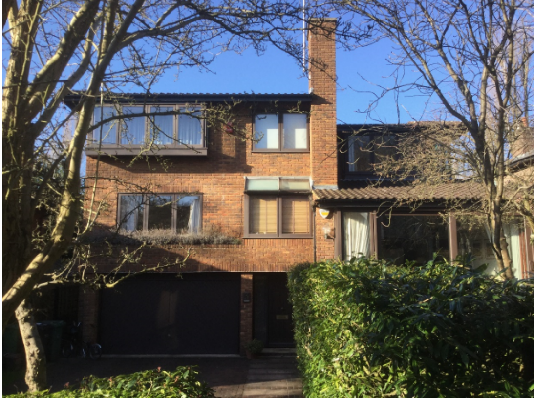
3. Front elevation of application site
