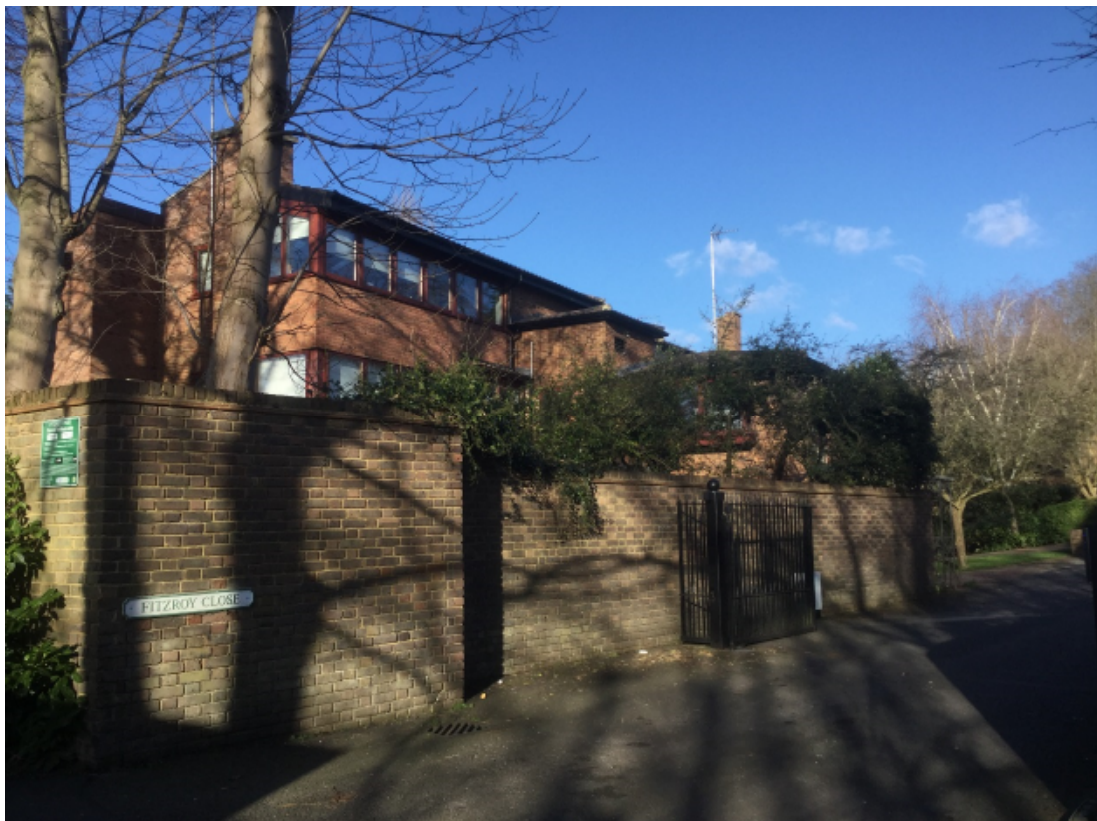
2. Entrance view within the close and neighbouring building at no. 4 Fitzroy Close
