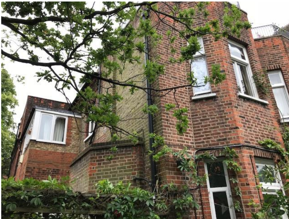
4. Side elevation of No. 3 Lyndhurst Gardens (Note bay window to be replaced by the proposals)
