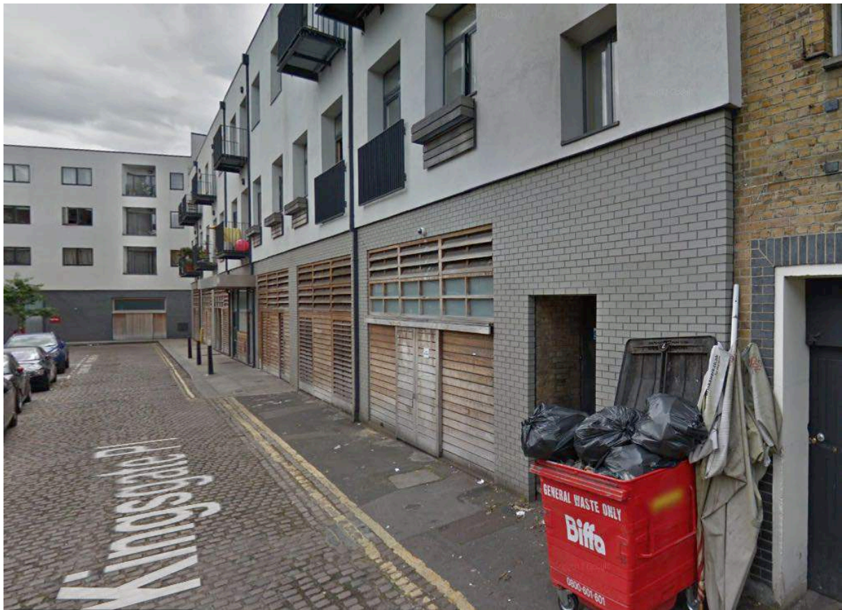
View of the location of the delivery entrance along Kingsgate Place
