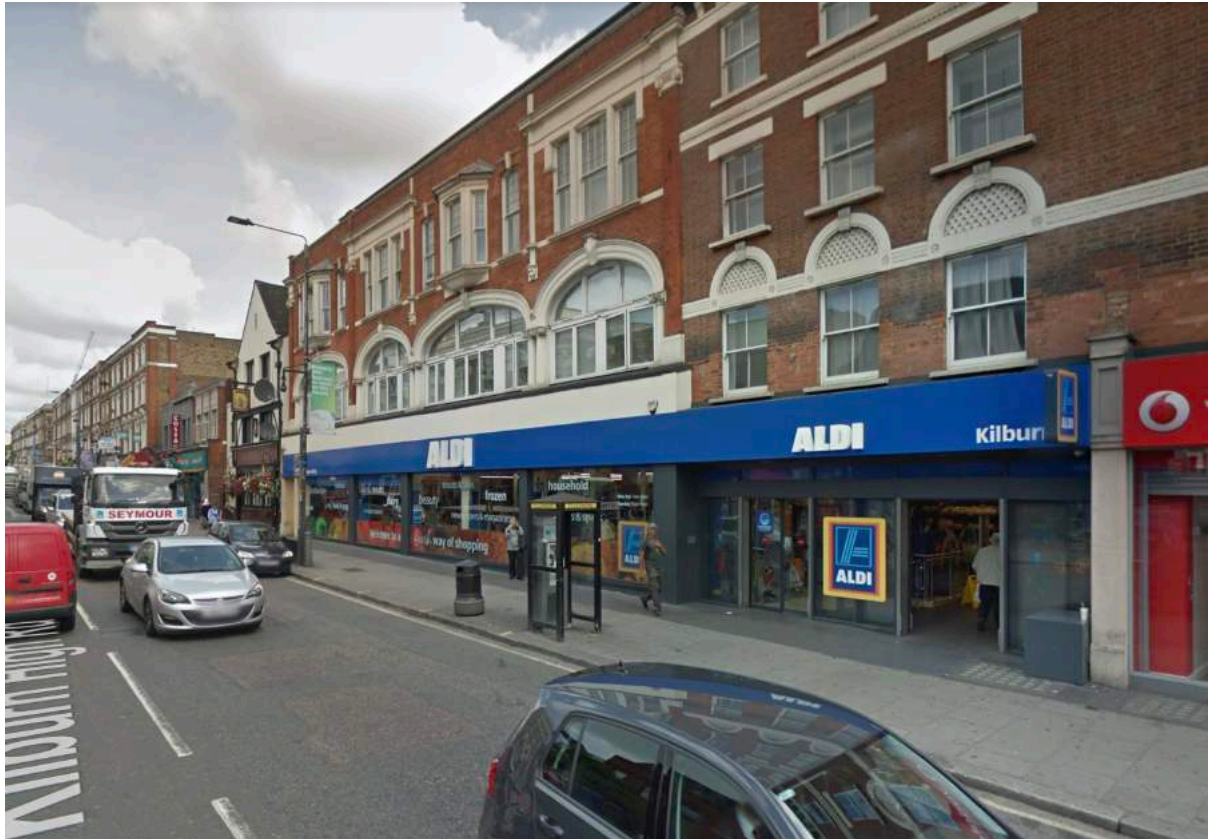
View of the existing Aldi store entrance along Kilburn High Road.
