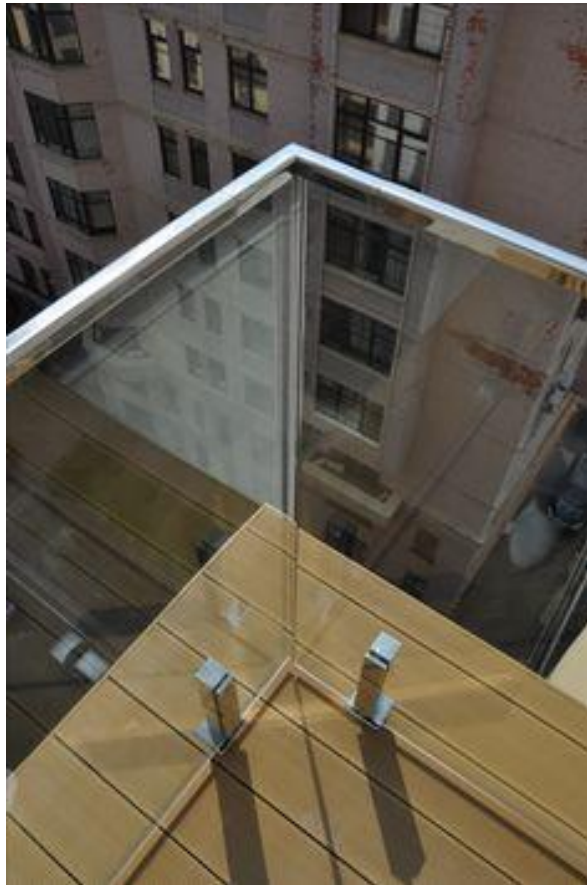
Glazed balustrade precedent (with base fixings)
