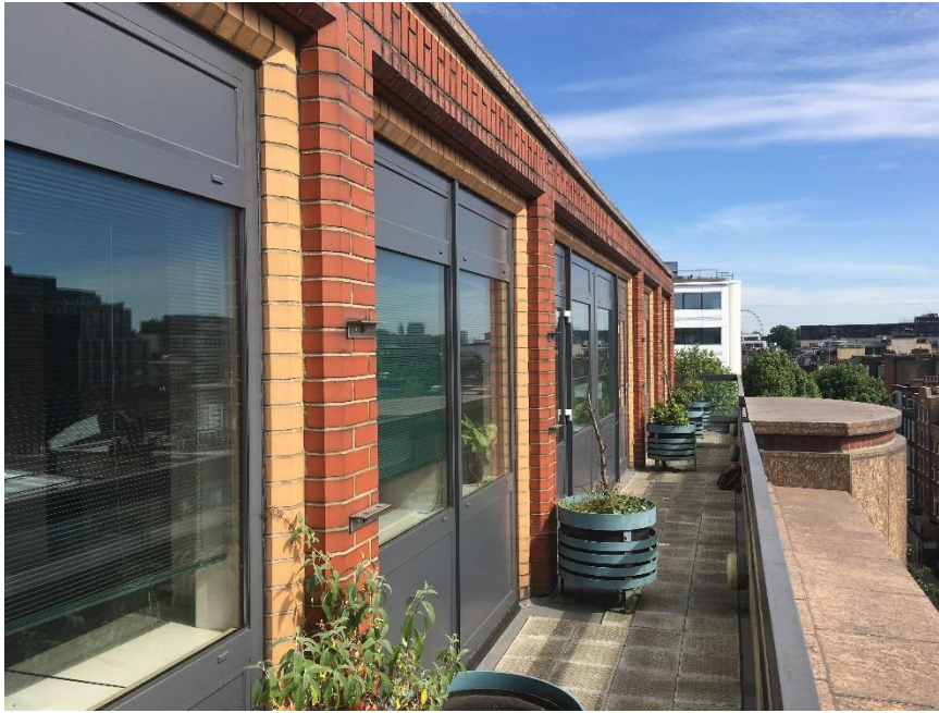
Photograph across existing balcony
