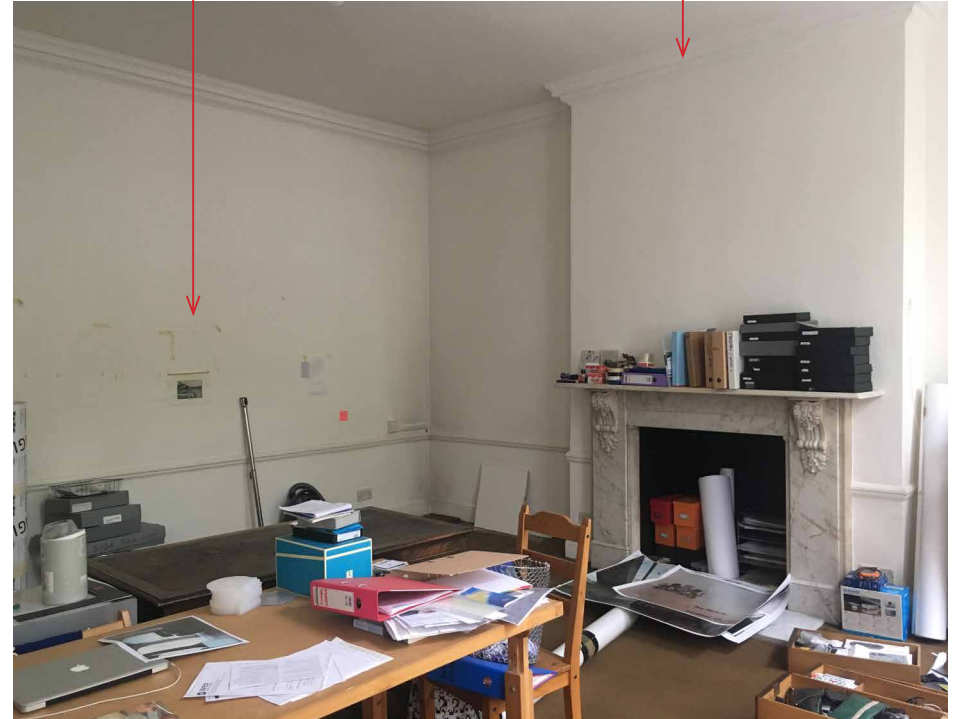
First Floor front Room View: Current April 2018
