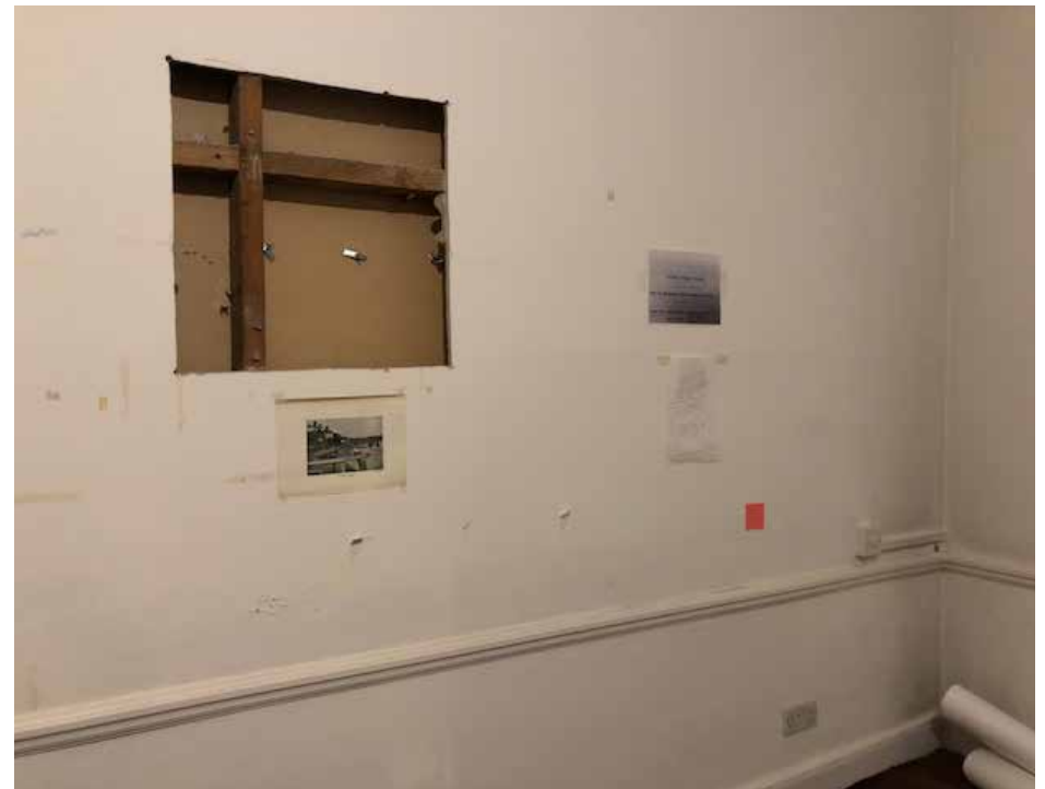
First Floor Front Room: Late addition infill timbers evident in opening
