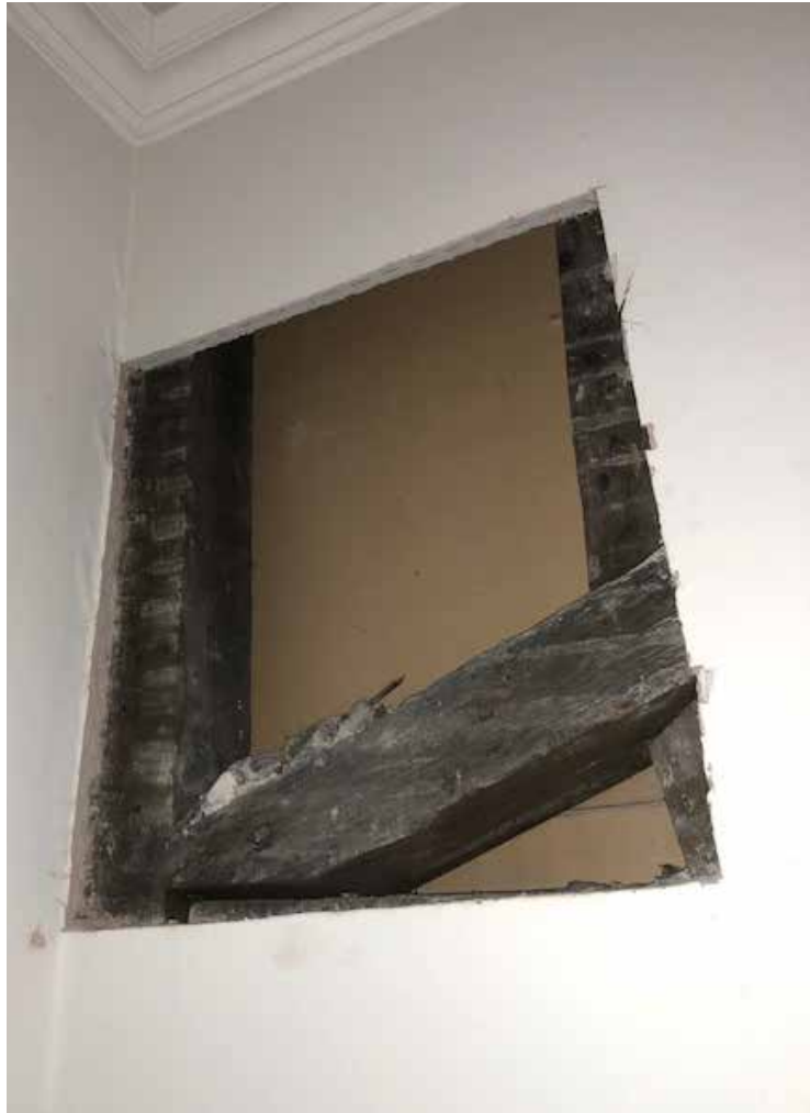
First Floor Front Room: Side Wall original timbers exposed
