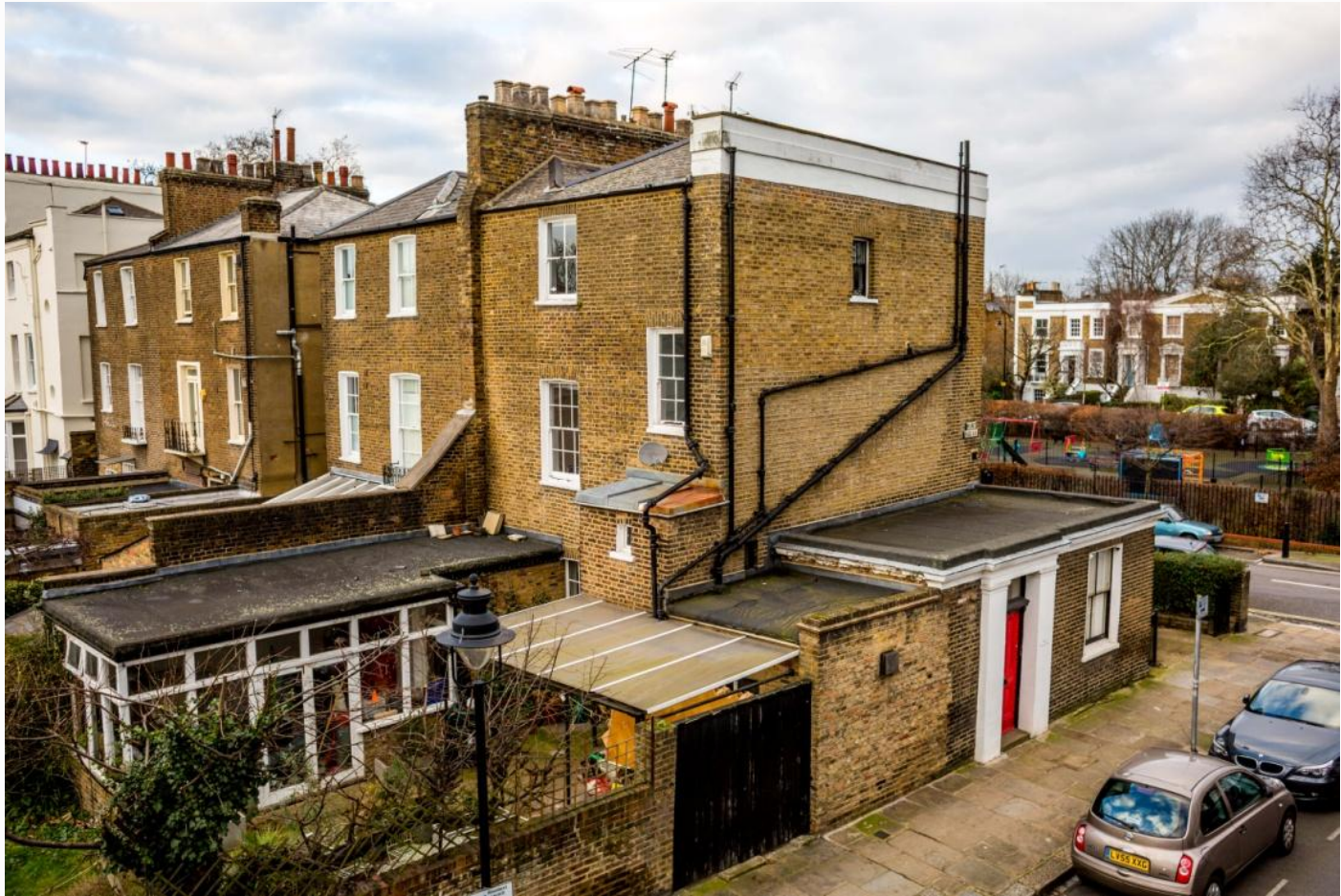
Fig 12 View of the rear and flank elevations of the building.
