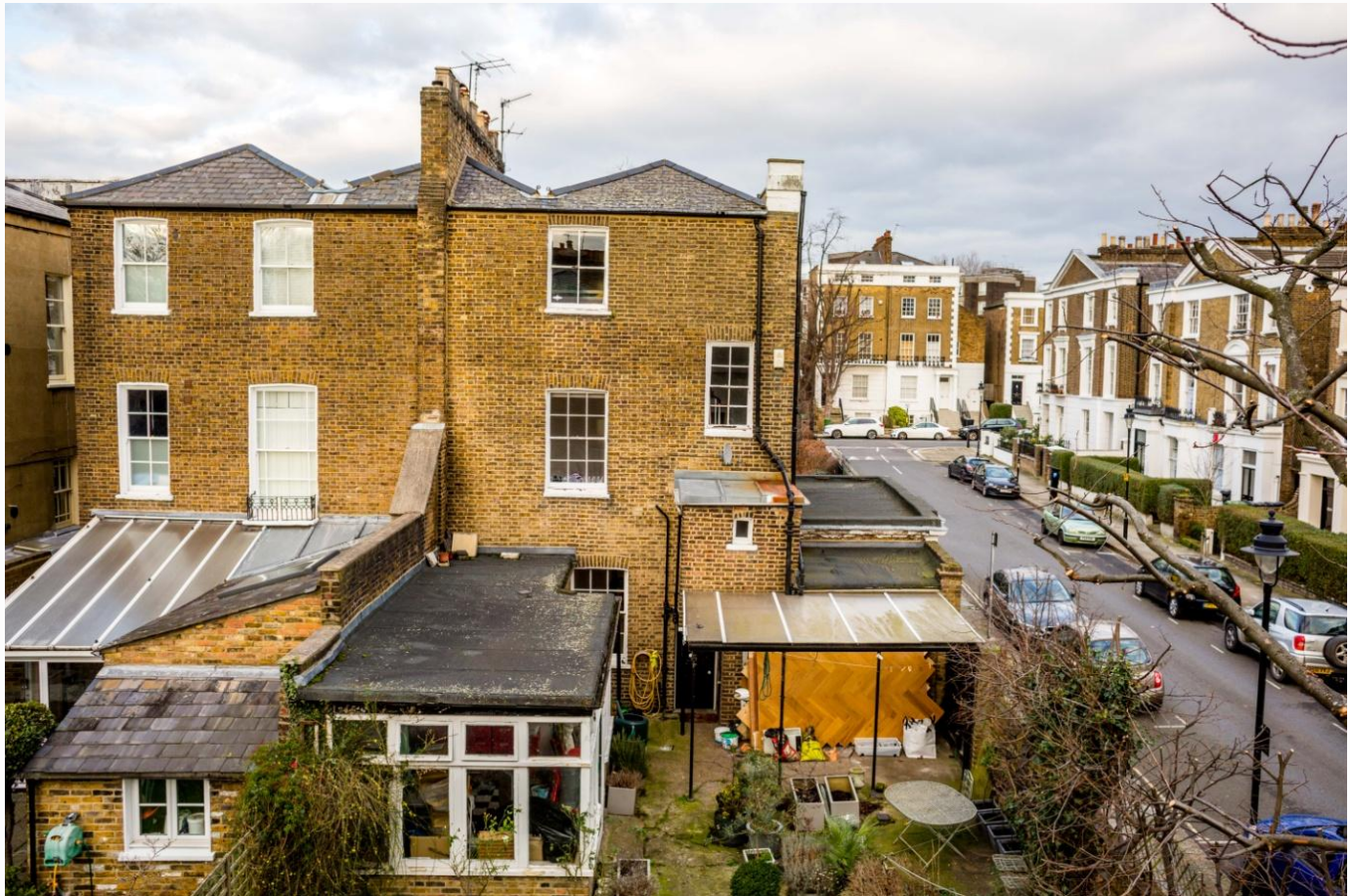
Fig 13 View of the rear elevation of the building.
