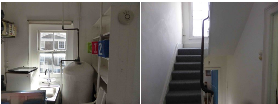
Figs. 6, 7 Existing side window second floor, existing stair window above current WC entry door
