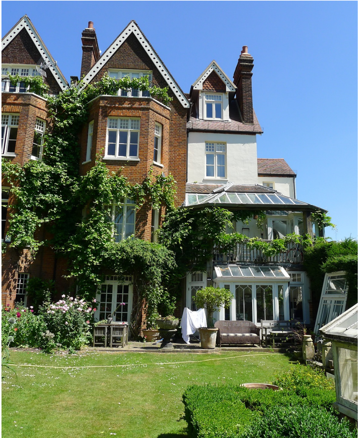
General view of rear from the garden
