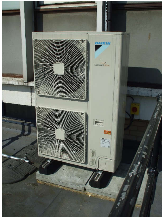
Figure A1: The new item of equipment (Daikin RZQG100L9V1 Outdoor unit)
