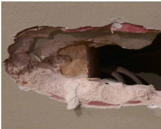
Exploratory works showing plasterboard partition wall between kitchen and front bedroom- no lath and plaster.
